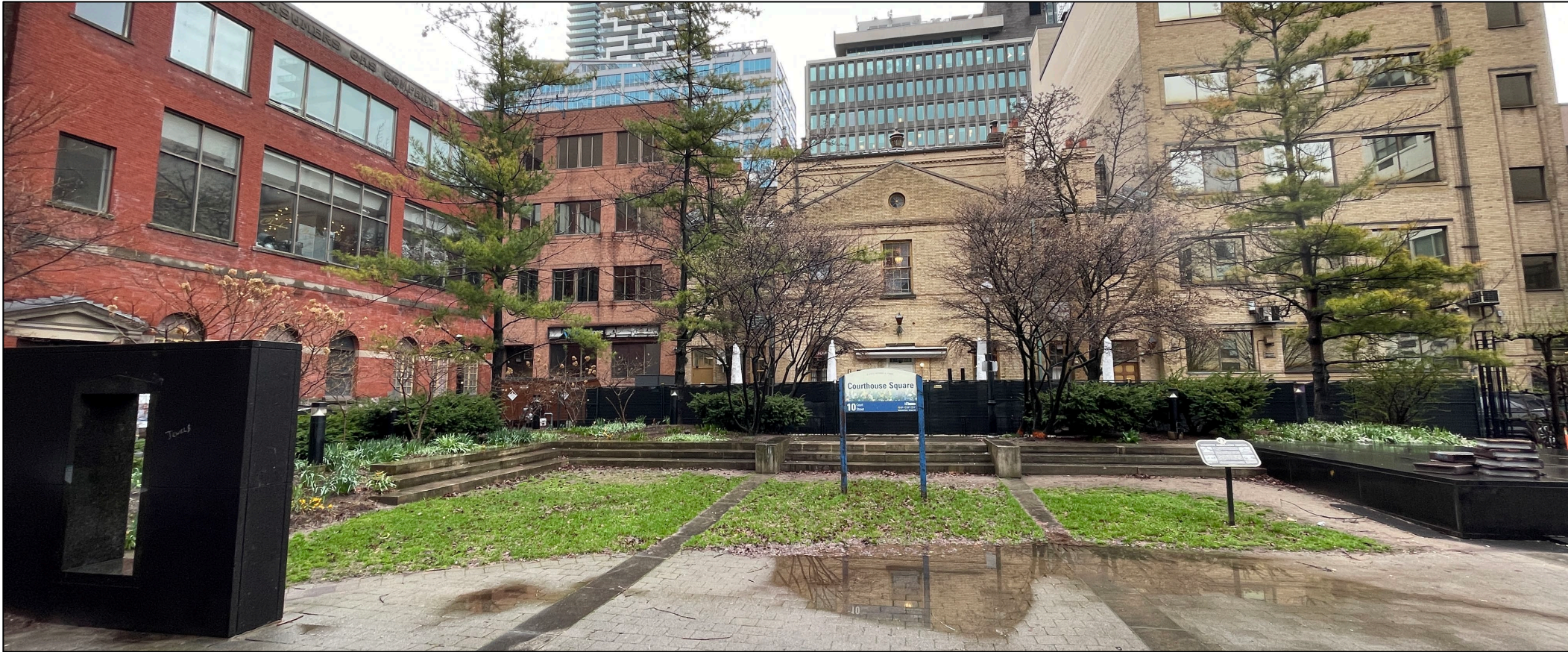
Rear elevations of 17-19 Toronto Street, 55 Adelaide Street East and 57 Adelaide Street East
