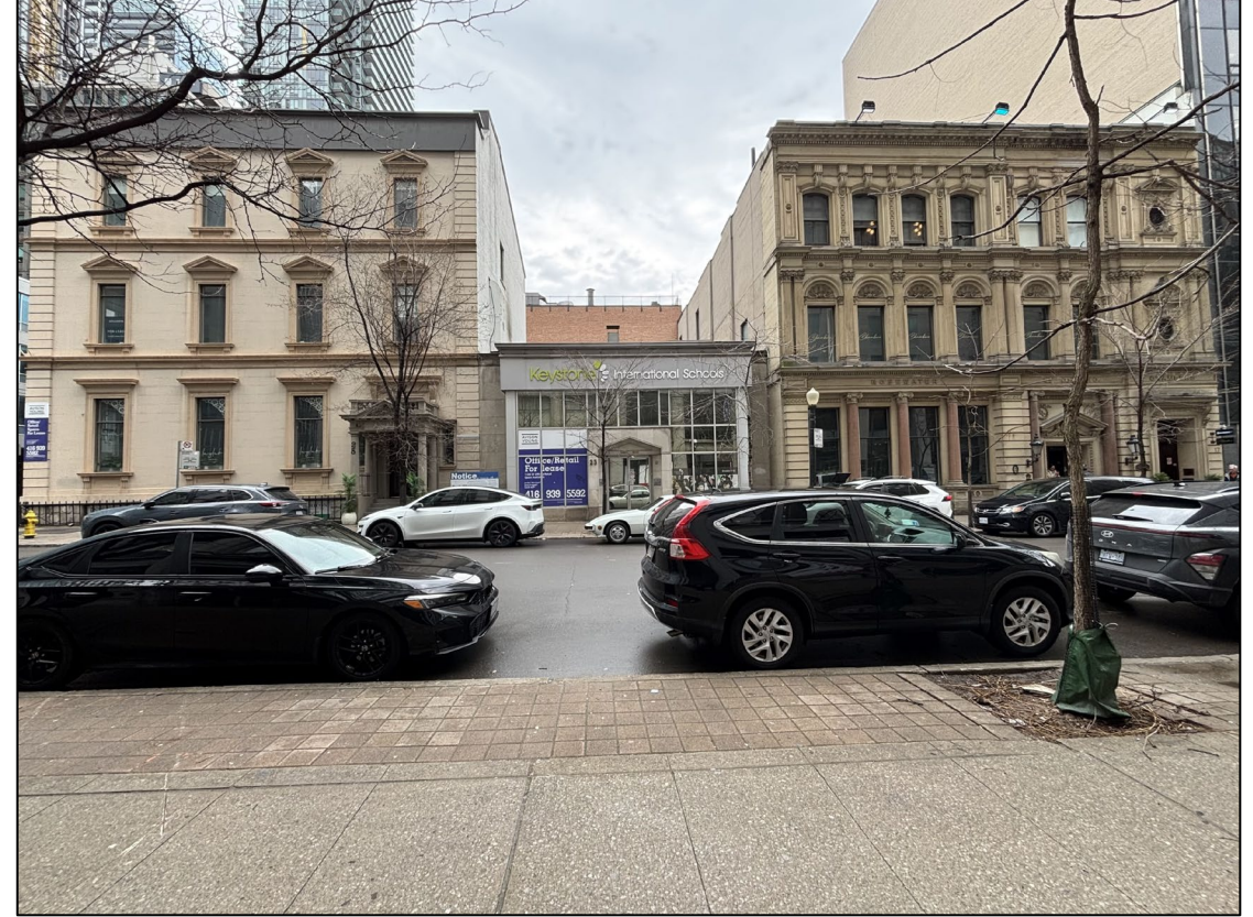
View of the north elevations of 25, 23, and 17-19 Toronto Street
