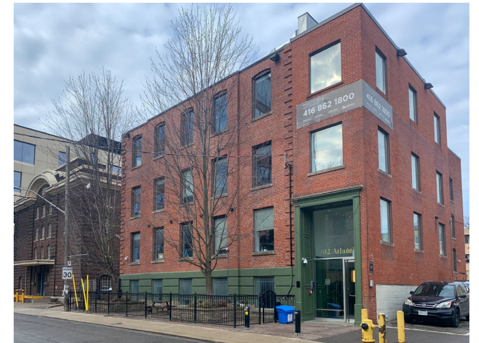
102 Atlantic Avenue, originally constructed for Sovereign Shoe Company c.1910 (Heritage Planning)
