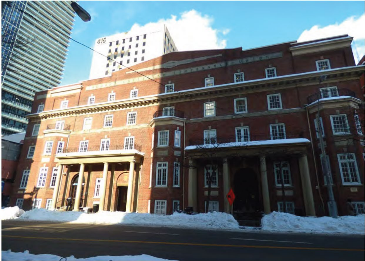
Figure 2: Primary (south) elevation of 20 Gerrard Street East (ERA Architects Inc., 2026).
