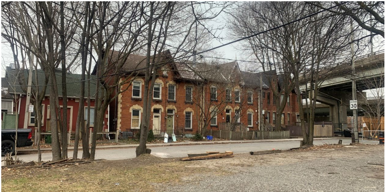
Figure 3: East (primary) elevations of the properties at 6-8 and 10-12 Sumach Street, and the south (side) elevation of 6-8 Sumach Street, looking northwest (Heritage Planning, 2025).
