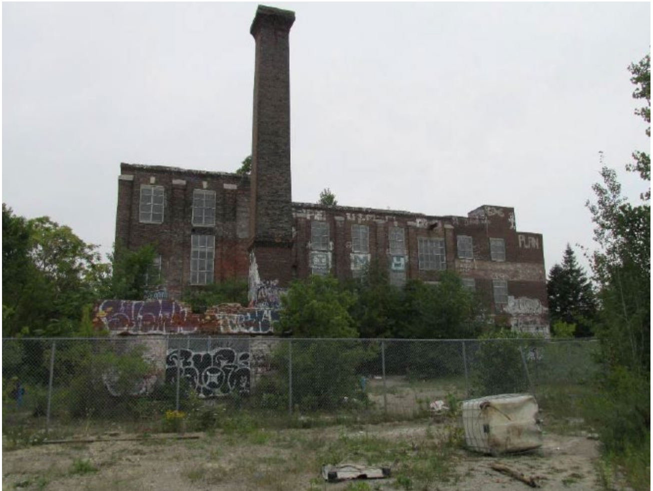
View of the east elevation, showing Building B and D, and C with its chimney stack at 40 Wabash Avenue (SBA, 2024).
