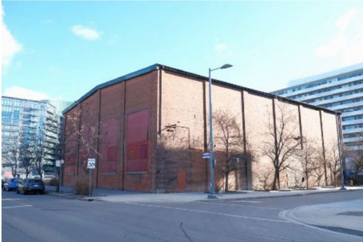
Figure 3: North and west elevation of 153 Eastern Avenue (Cleaning Room building), looking southeast (Philip Goldsmith Architect, 2025).
