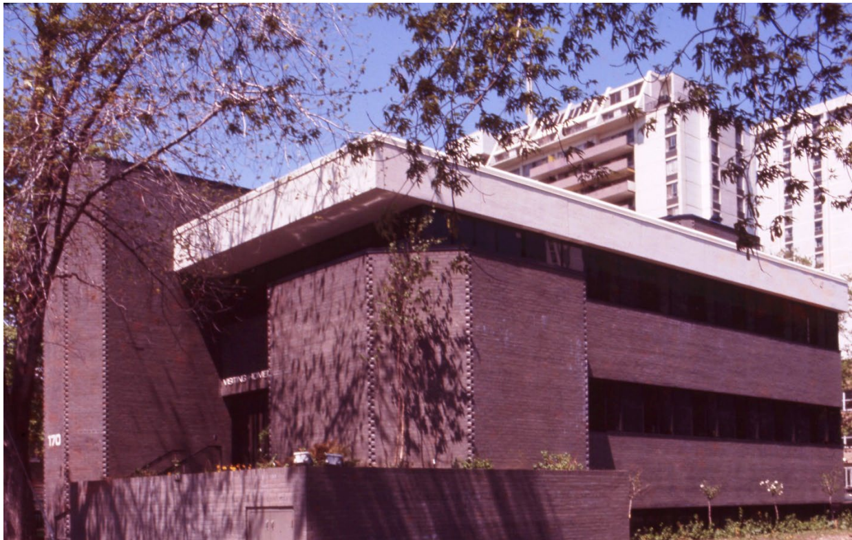
Early photograph of the VHA building, showing the principal (south) and side (east) elevations with original pigmented concrete brick (Leslie Rebanks)
