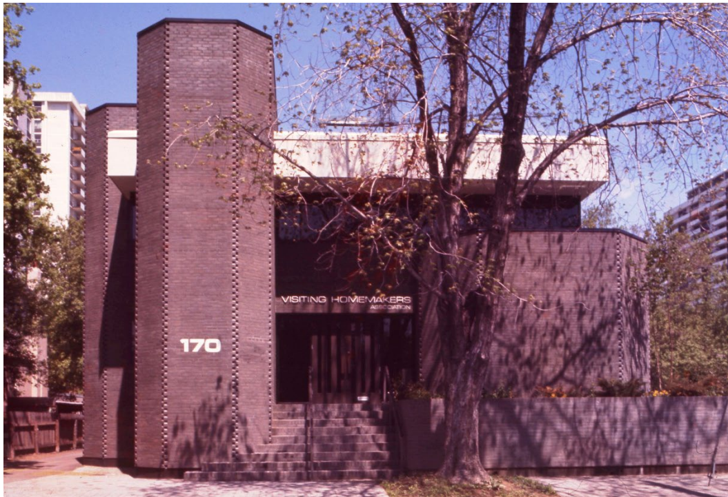
Early photograph of the VHA building showing the original pigment of the concrete brick cladding and paving (Leslie Rebanks)
