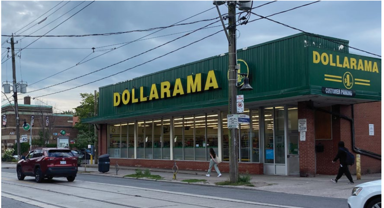
North elevation of the existing building at 1337 Queen Street West (ERA Architects Inc., 2026).
