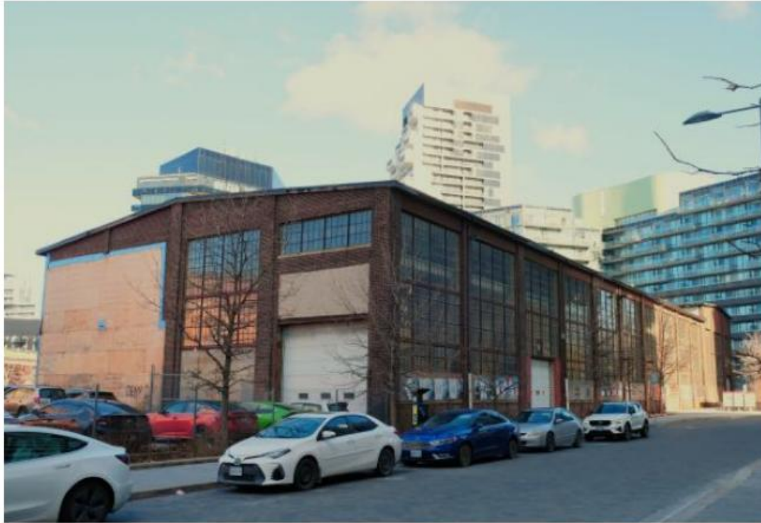
South and west elevation of 185 Eastern Avenue (Machine Shop building), looking northeast (Philip Goldsmith Architect, 2025).
