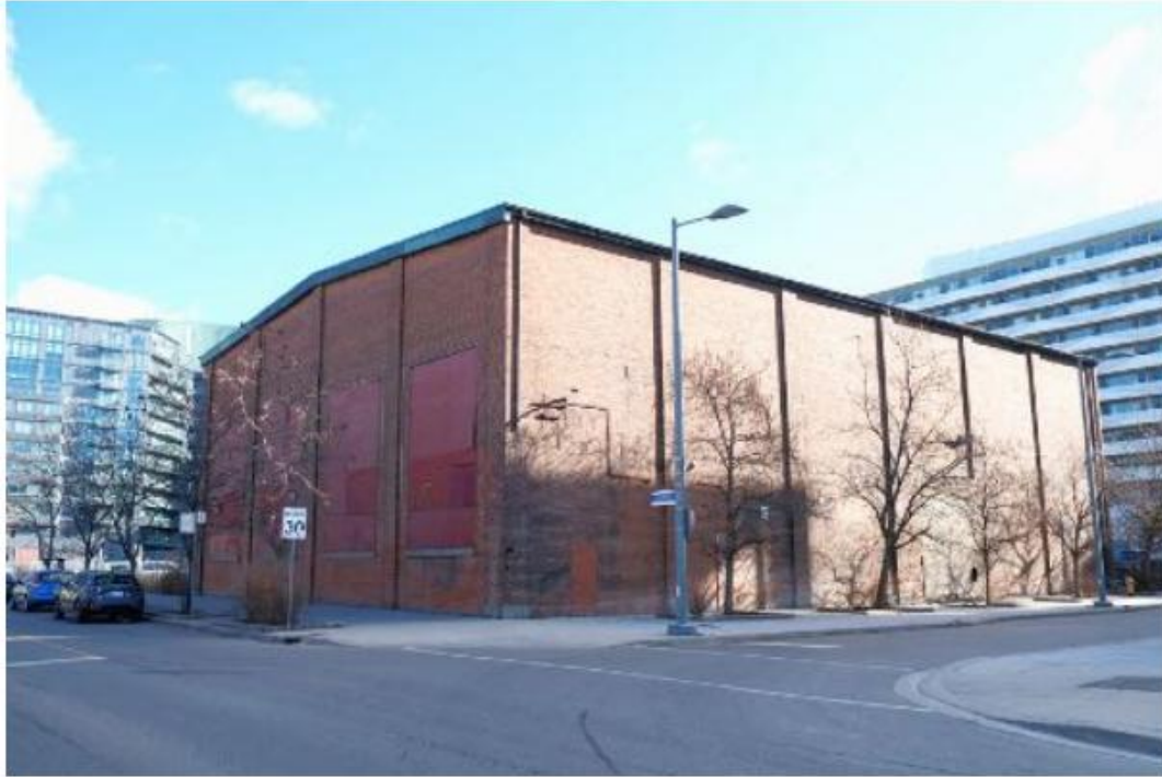
North and west elevation of 153 Eastern Avenue (Cleaning Room building), looking southeast (Philip Goldsmith Architect, 2025).
