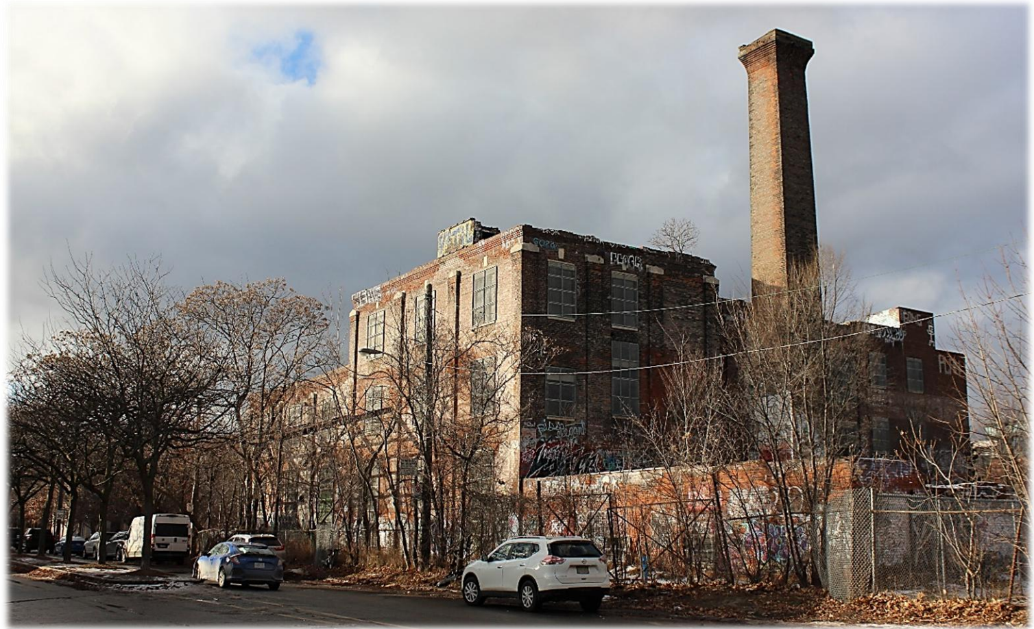
View of the southeast elevation of 40 Wabash Avenue looking northwest from Wabash Avenue (City of Toronto, 2025).
