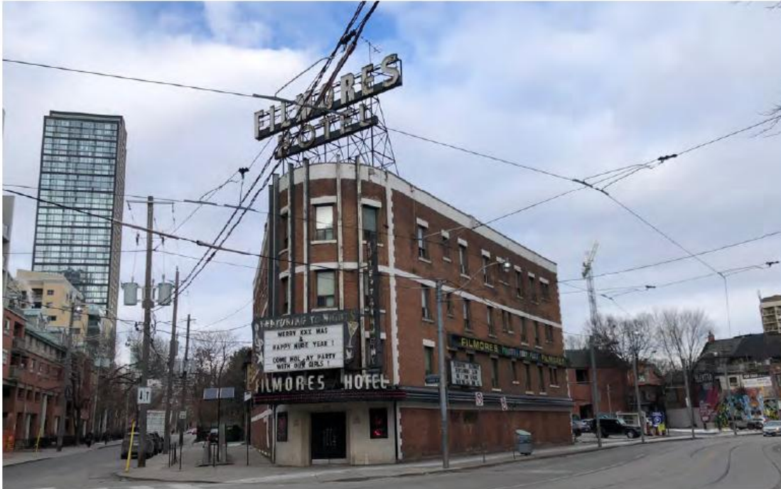
Photo of the south elevation of the existing building at 212 Dundas Street East (Giaino + Associates Architects Inc., 2025).
