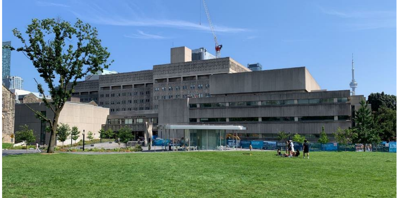
The Medical Sciences Building complex at 1 King's College Circle, north elevation as viewed from King's College Circle lawn, looking southeast (Heritage Planning, 2025).
