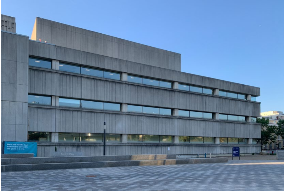
North elevation of Wing B, looking southwest (Heritage Planning, 2025).
