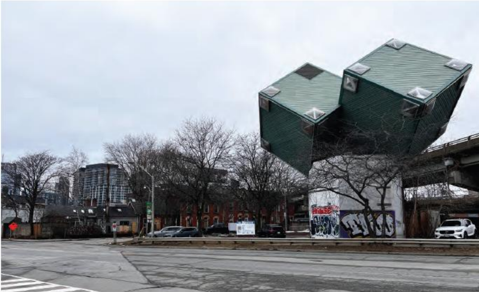
View of 1 Sumach Street, also showing the east (primary) elevations of 6-8 and 10-12 Sumach Street, looking northwest (ERA Architects Inc., 2026).
