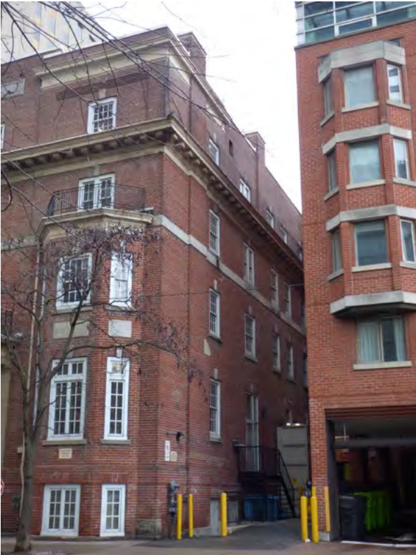
Partial east elevation of 20 Gerrard Street East (Source: ERA, January 2026).
