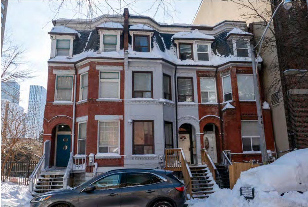
23-27 McGill Street, north façade (Source: ERA, 2026).
