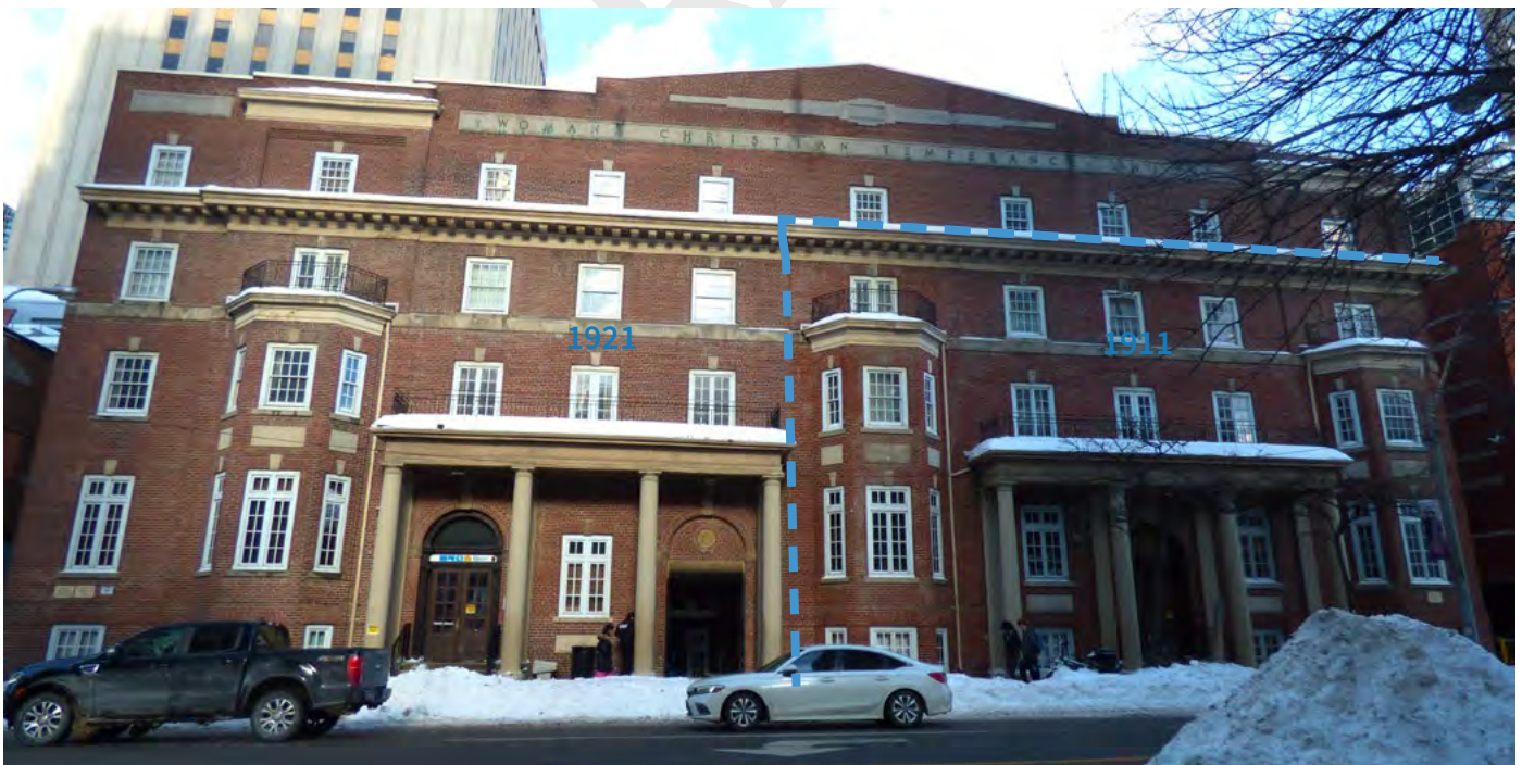
1. Overall front (south) elevation of 20 Gerrard St E showing 1911 and 1921 phases of construction (ERA, January 2026)
