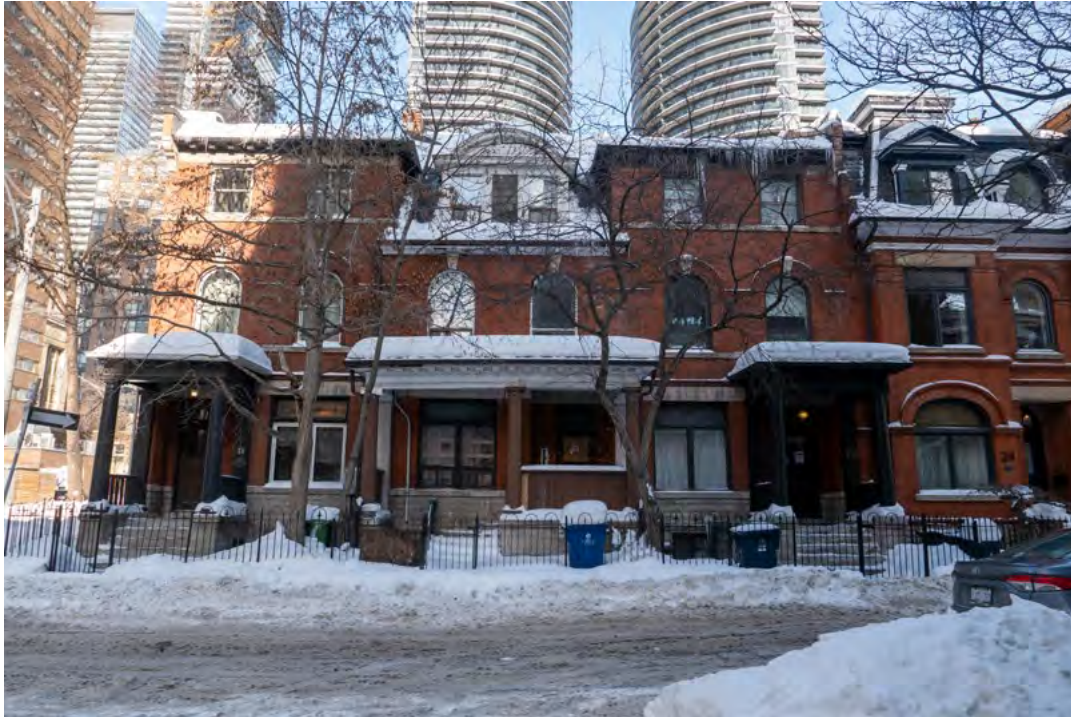
18-22 McGill Street, south façade (Source: ERA, 2026).
