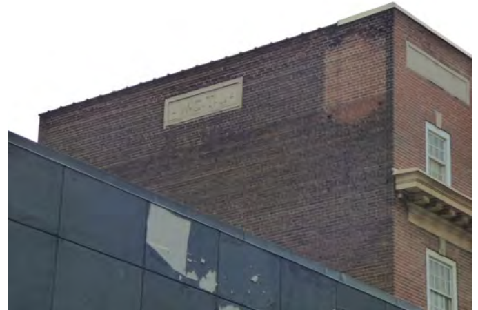
40. West elevation, visible above adjacent building (ERA, December 2025)
