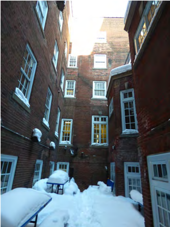
Interior court space of 20 Gerrard Street East (ERA, January 2026).
