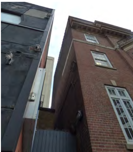
42. Portion of west elevation partially concealed by neighbouring building (ERA, December 2025)
