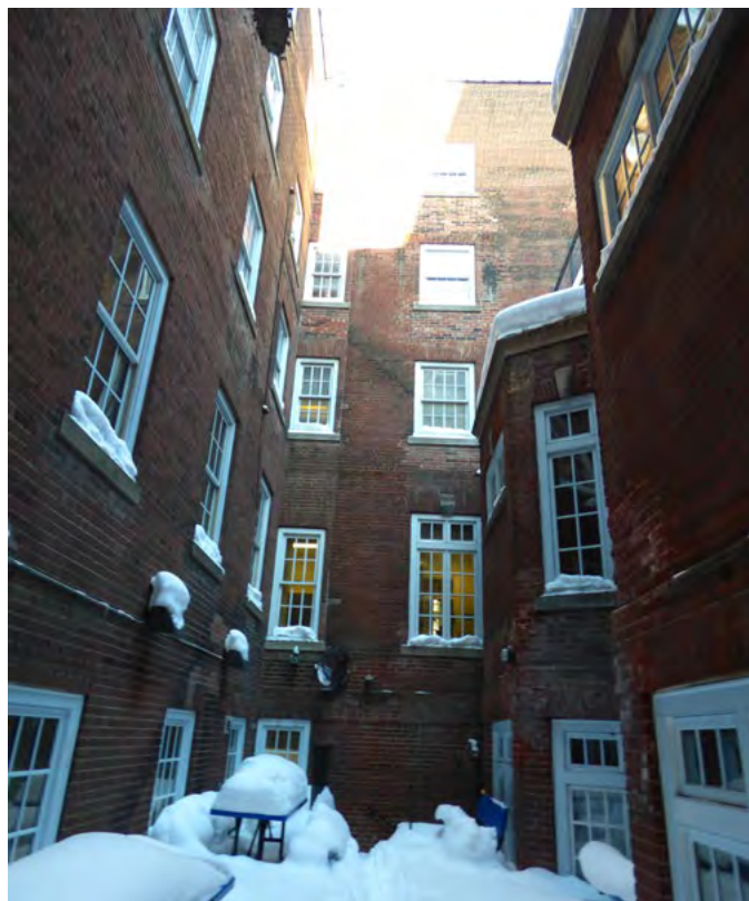
Interior court space of 20 Gerrard Street East (ERA, January 2026).
