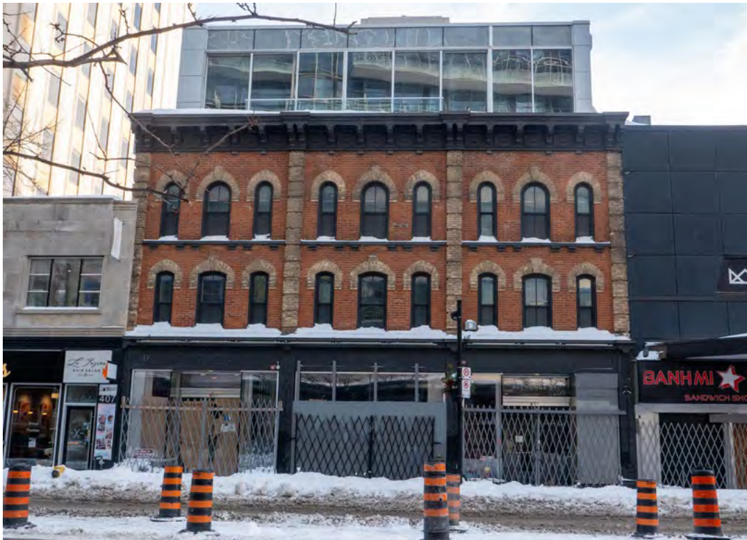
401-405A Yonge Street, west façade (Source: ERA, 2026).
