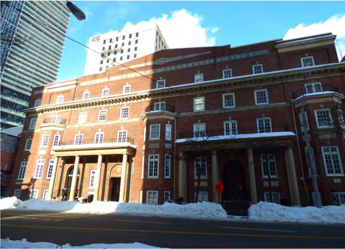
South (primary) façade of 20 Gerrard Street East (Source: ERA, January 2026).
