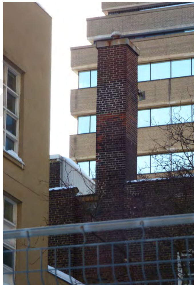
46. Chimney at North Elevation (ERA, January 2026)
