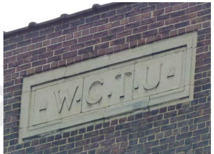
41. Artificial stone signage from 1911, relocated to the west elevation in 1921 (ERA, December 2025)
