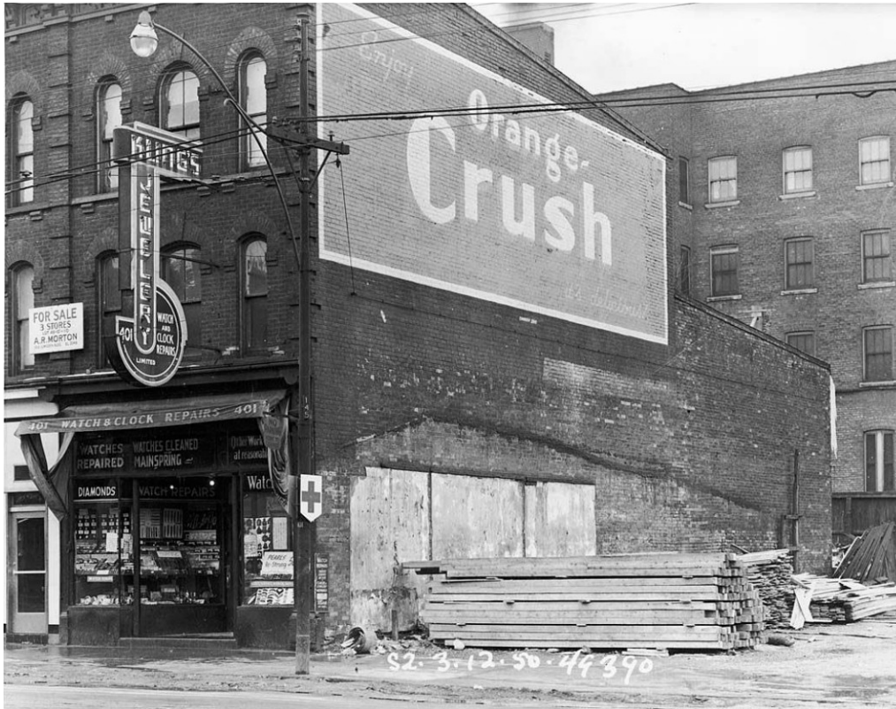
South-west corner 401 Yonge Street in 1950 (Source: City of Toronto Archives).
