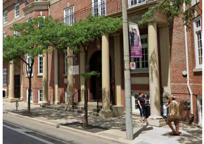
Current inaccessible entrance at east portico, 20 Gerrard Street East (GoogleMaps, 2024).
