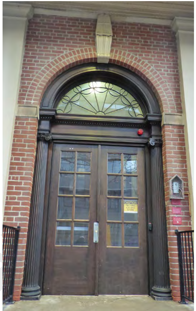
22. East entrance door (ERA, December 2025)
