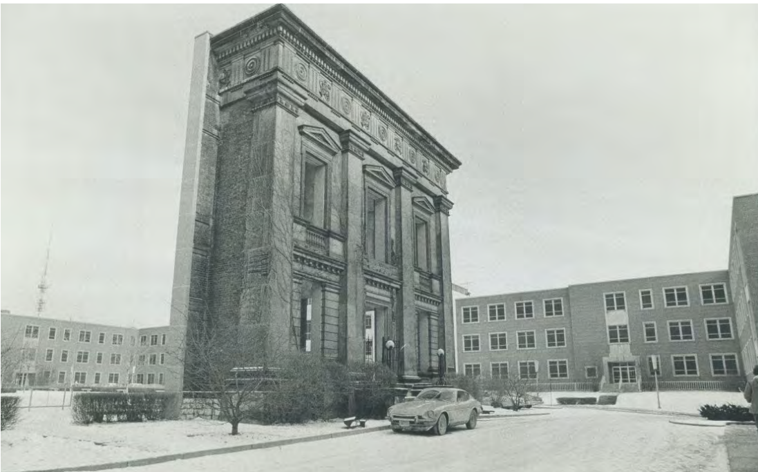
Remnant façade of the Normal School in 1975, within Kerr Hall quadrangle (Source: Toronto Public Library Digital Archive).
