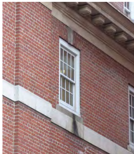
38. Third-floor window east elevation (ERA, December 2025)
