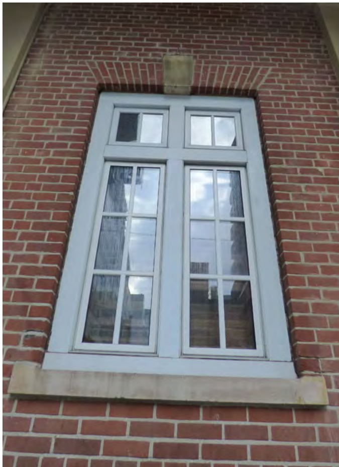
26. Typical condition of ground floor window (ERA, December 2025)
