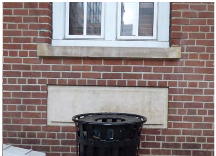
12. Condition of natural stone accents within portico area (ERA, December 2025)
