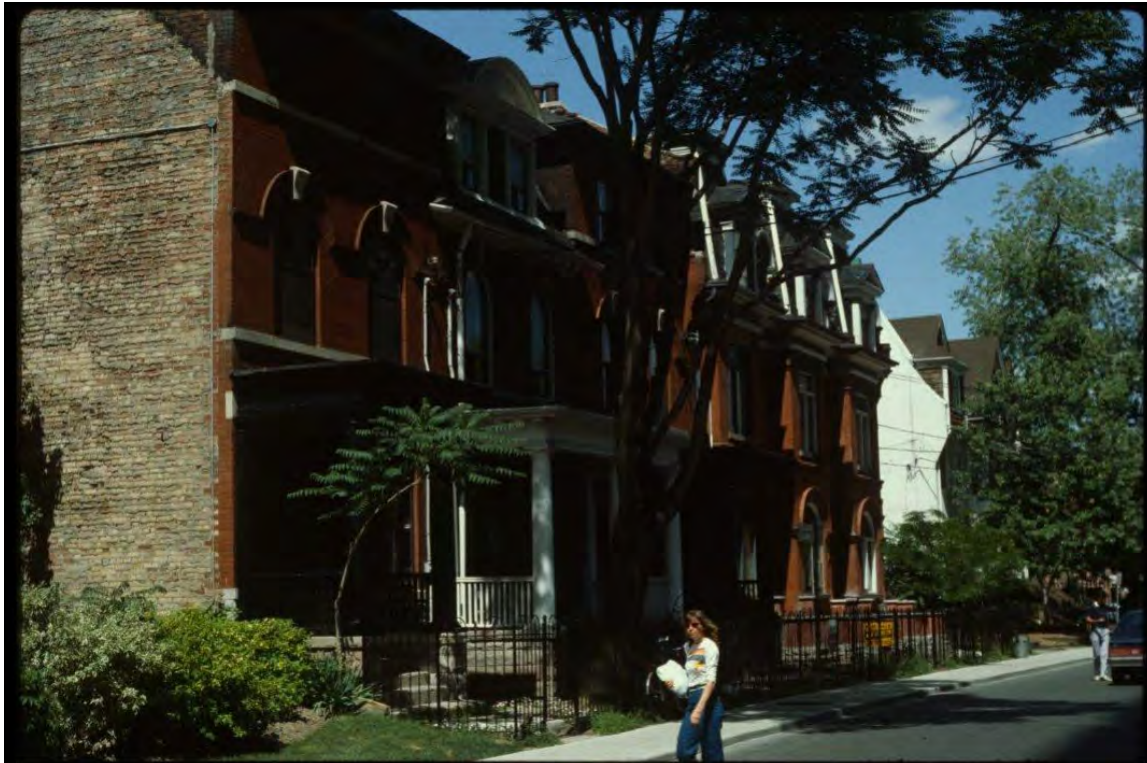
View of 18 to 28 McGill Street row housing c. 1986-1992 (Source: City of Toronto Archives).
