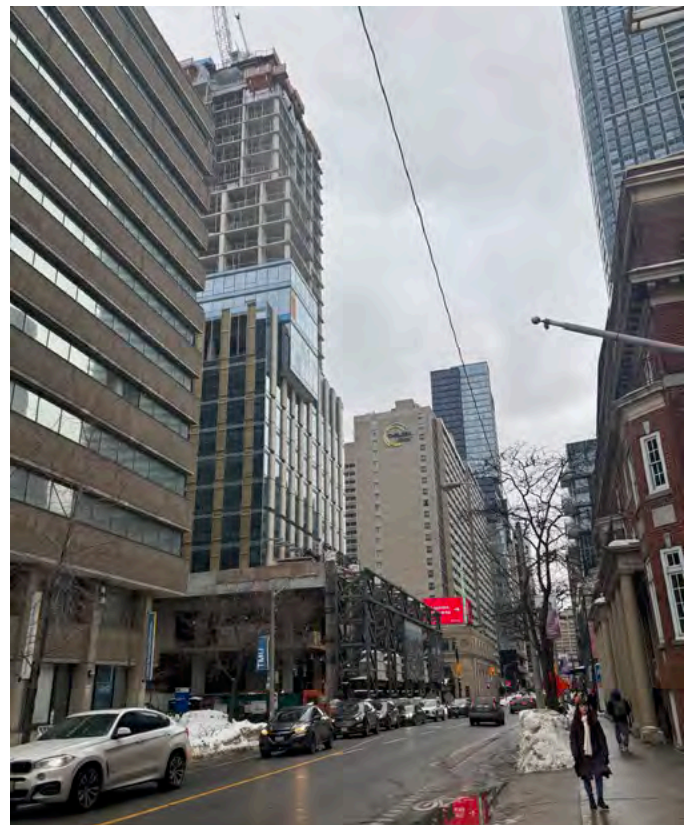
Context view looking west along Gerrard Street (ERA, February 2026).
