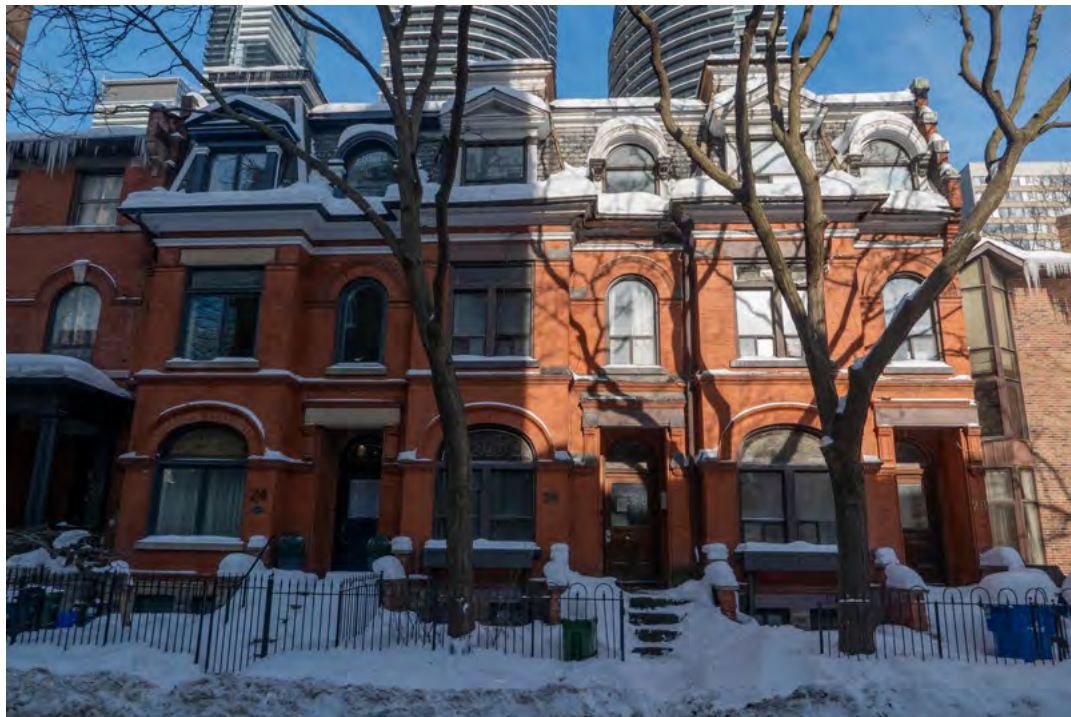
24-28 McGill Street, south façade (Source: ERA, 2026).
