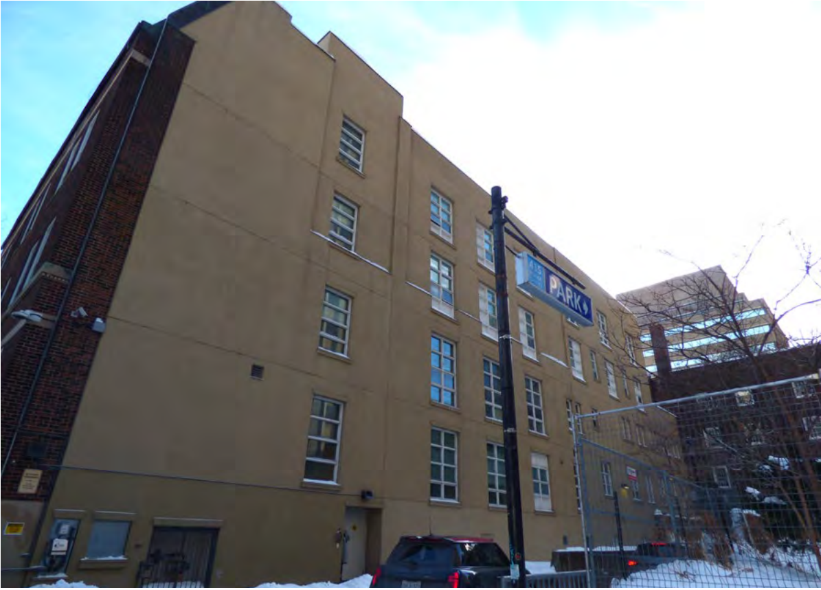
West elevation of 21 McGill Street (ERA, January 2026).
