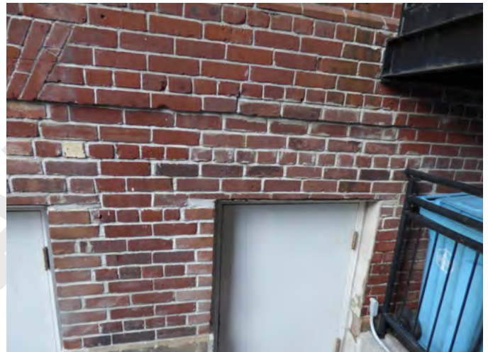
36. Modifications at added basement doors, east elevation (ERA, December 2025)
