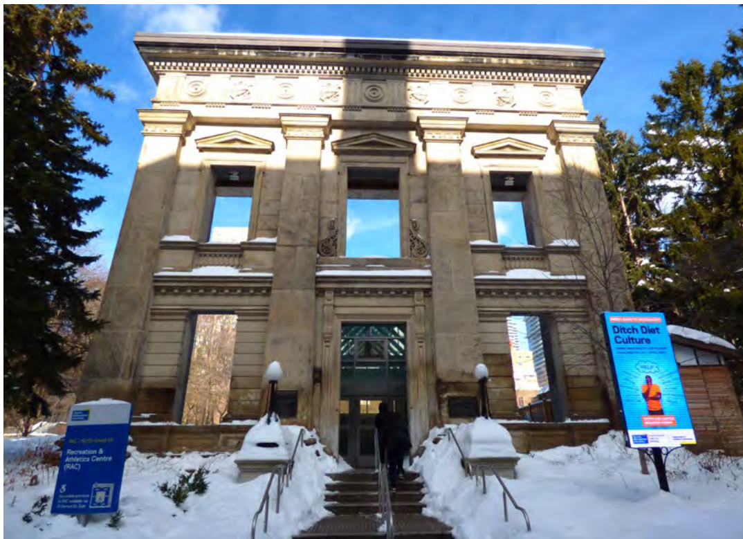
Remnant façade from the Normal School. The school was constructed at 21, 31-33 Gerrard Street East, then relocated in the 1940s and demolished in 1963. The remaining portion of the façade is located within the Kerr Hall quadrangle at 50 Gould Street (Source: ERA, 2026).
