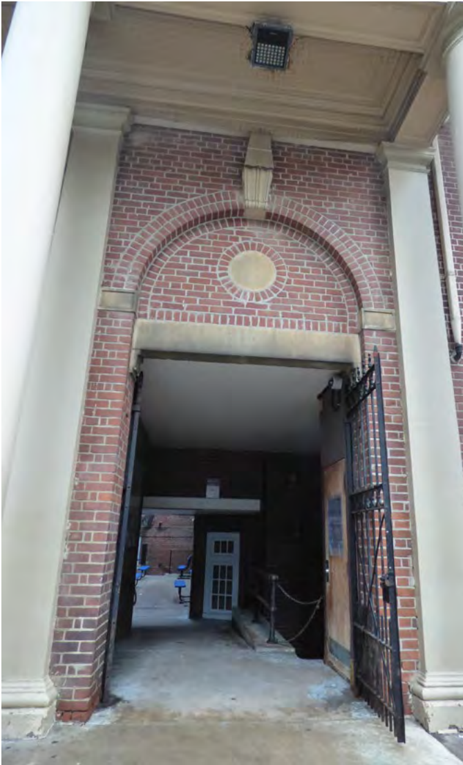
15. Brick and natural stone masonry at entrance to interior court space (ERA, December 2025)
