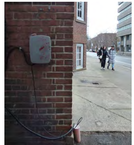
44. Previous rebuilding at base of southwest corner (ERA, December 2025)
