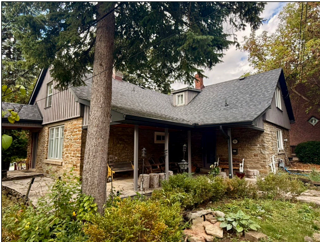
Figure 2. 34 Jason Road, southeast façade (Alex Corey, September 2025).
