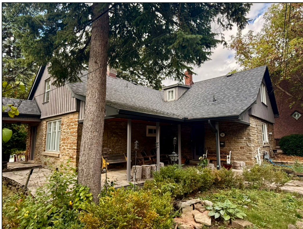
Figure 3. 34 Jason Road, southeast façade (Alex Corey, September 2025).
