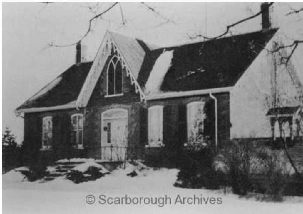
Figure 4. Photograph of the north (front) facade of the Wheler House, date unknown. Scarborough Historical Society.
