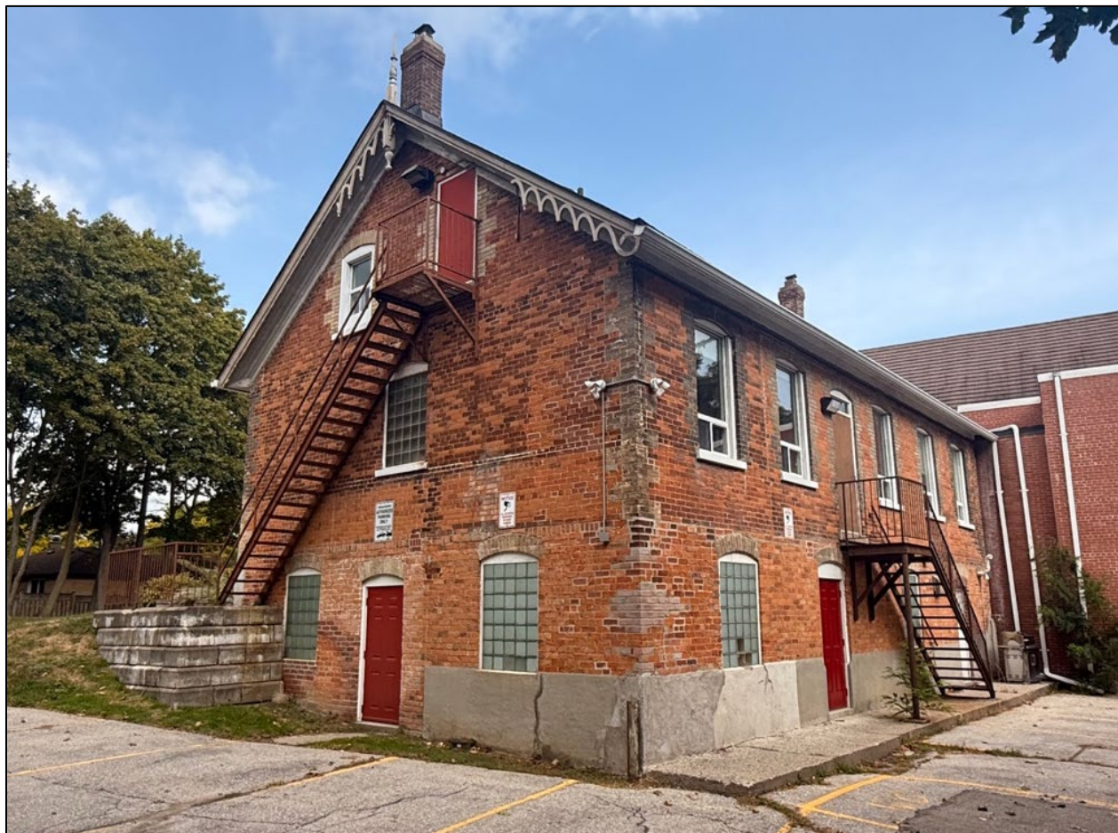
Figure 3. 328 Bellamy Road North, J.P. Wheler House (Alex Corey, September 2025).
