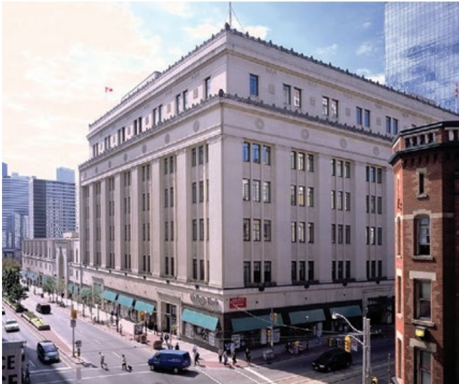
College Park looking southwest at the corner of Yonge Street and College Street
