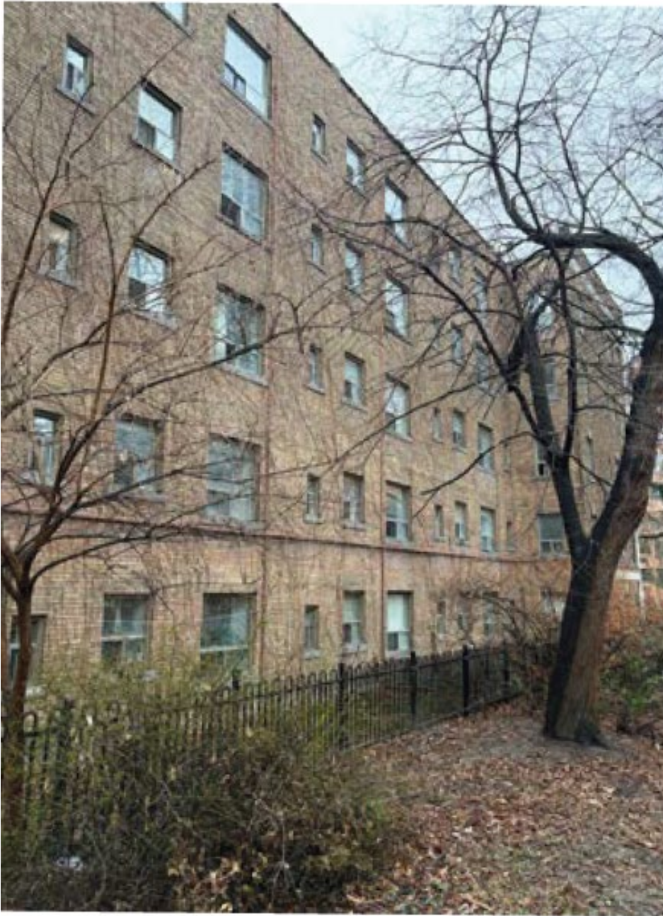
Figure 3: Portion of the side (west) elevation of 64 Wellesley Street East, looking southeast (ERA Architects Inc., 2026).
