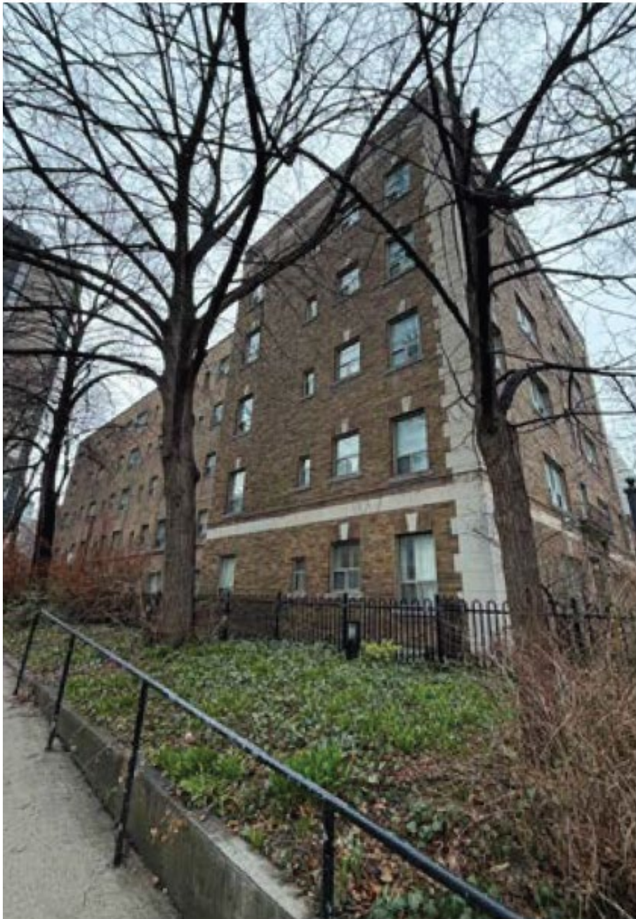
Figure 4: Side (west) and the primary (south) elevation of 64 Wellesley Street East, looking northeast (ERA Architects Inc., 2026).
