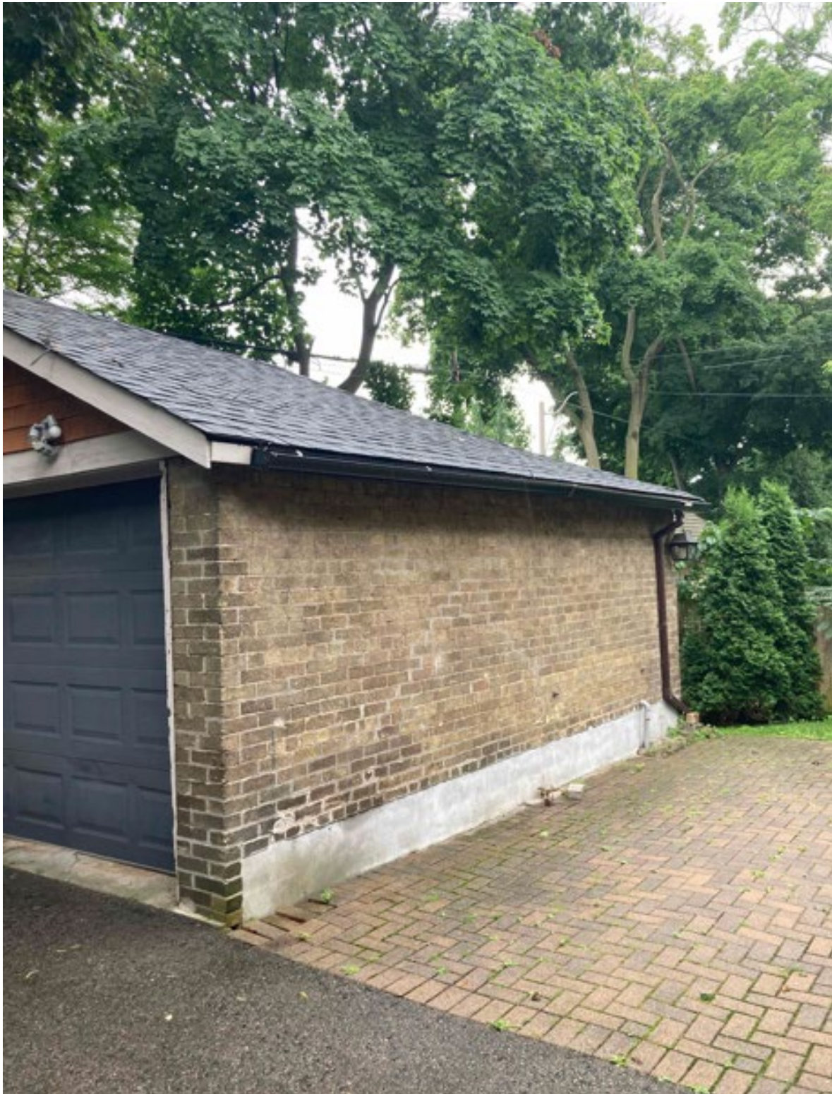
Photo of existing detached garage at 79 Whitehall Road, taken from the rear yard (Christopher Walker Architect, 2025).
