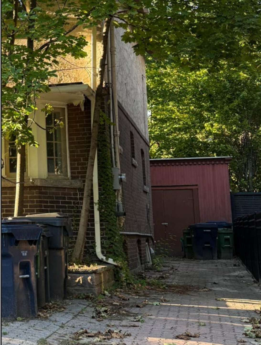
View of the south elevation at 162 Douglas Drive, showing the principal residence and existing detached garage (House Lab Inc, 2025).
