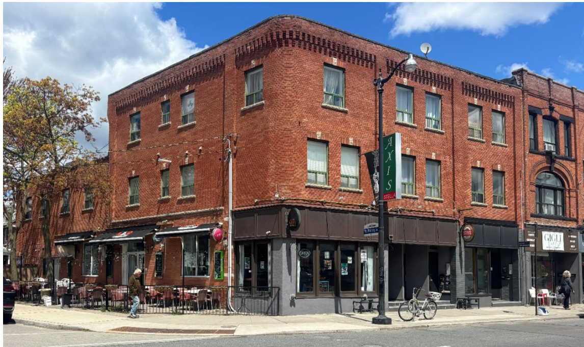
3044 Dundas Street West, principle (south) and west elevations as viewed from the southwest (City of Toronto Heritage Planning, 2026)
