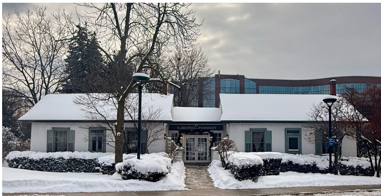
Figure 3. 4150 Yonge Street, north façade (Alex Corey, January 2026).
