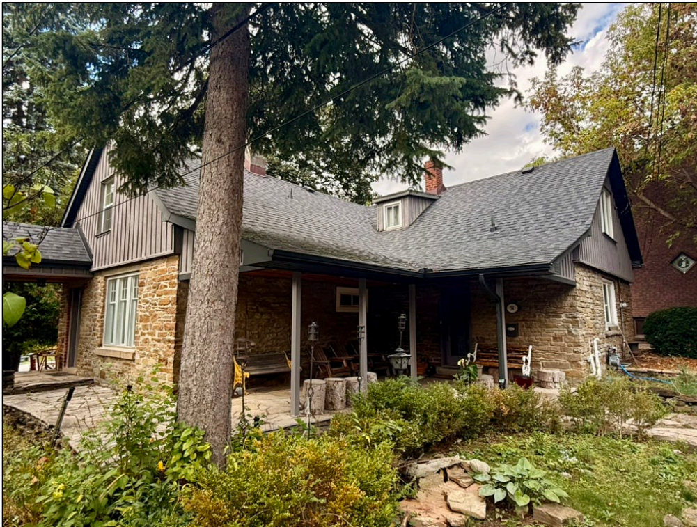
Figure 10: 34 Jason Road, southeast façade (Alex Corey, September 2025).
