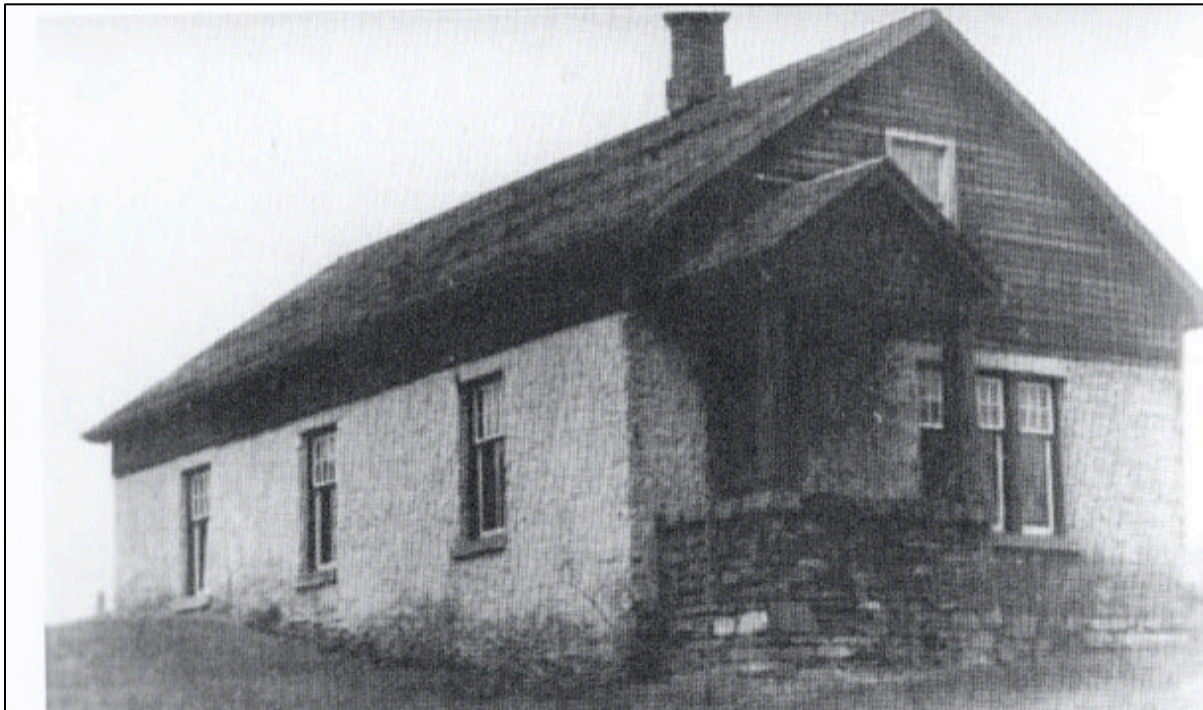
Figure 6: 34 Jason Road, date unknown (pre-1926). Note the stucco cladding, which was subsequently removed. Twitchin, The History of Thistle Town.
