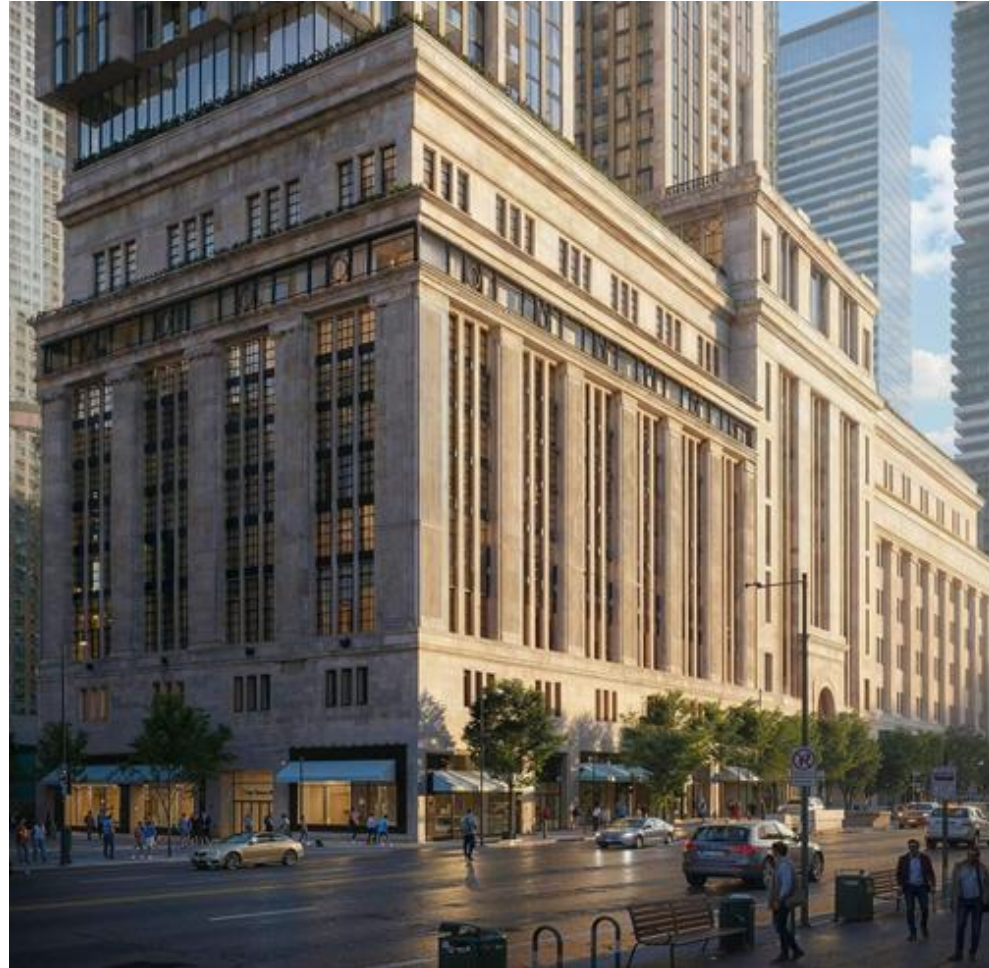
Looking Northwest at South and East (Yonge St) Facades
