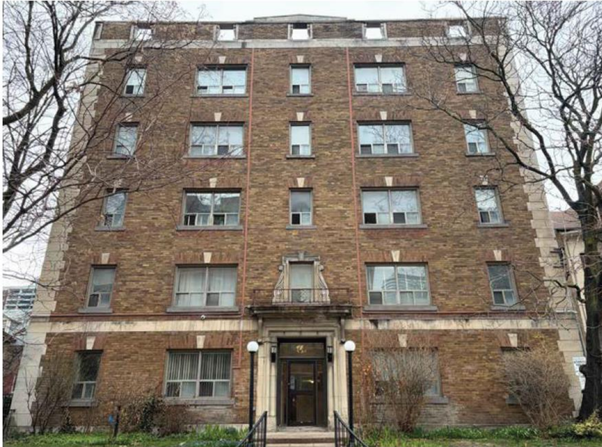
Primary (south) elevation of 64 Wellesley Street East, looking north (ERA Architects Inc., 2026).
