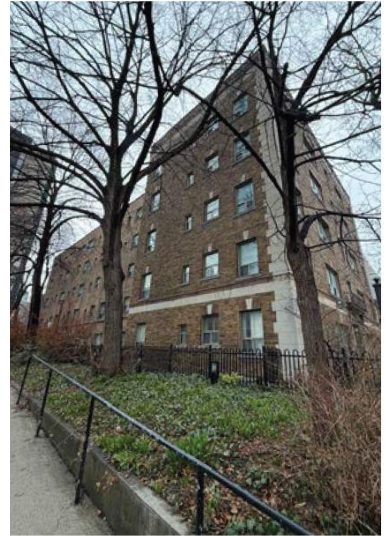
Side (west) and the primary (south) elevation of 64 Wellesley Street East, looking northeast (ERA Architects Inc., 2026).
