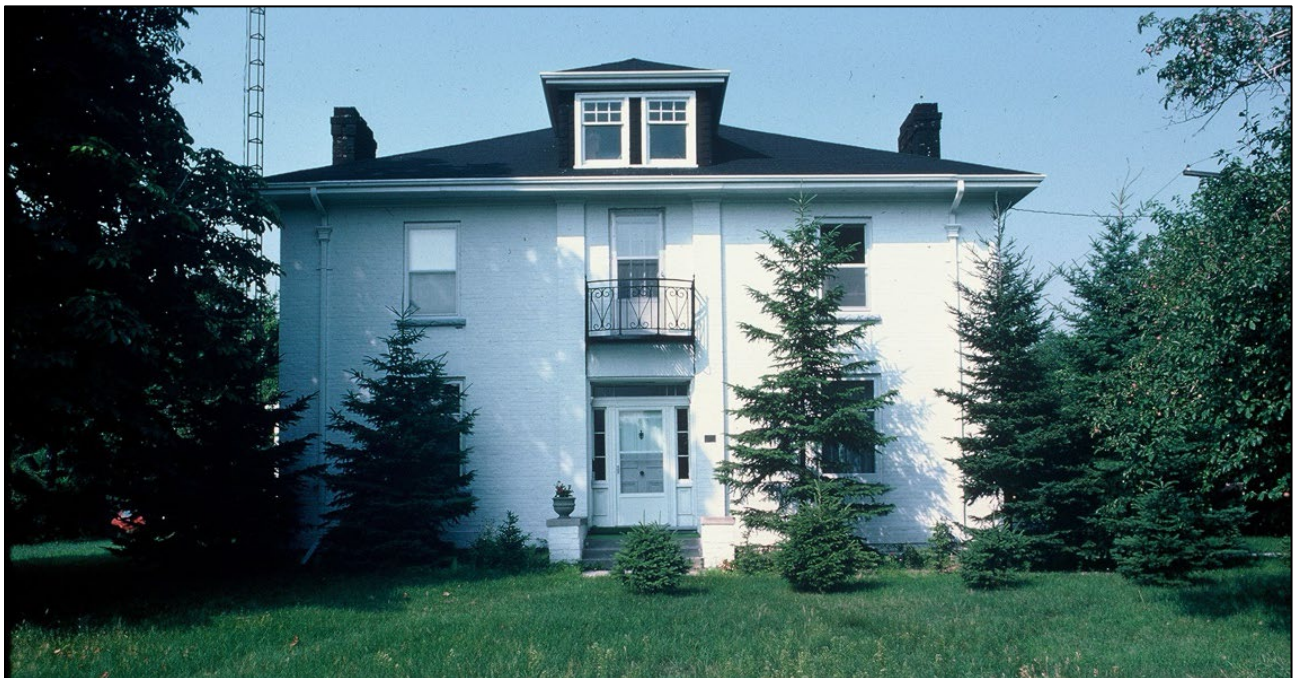
Figure 13. 7 Meadowcrest Road (formerly 848 Royal York Road), primary (east) façade detail. Date Unknown. Toronto Historical Board.
