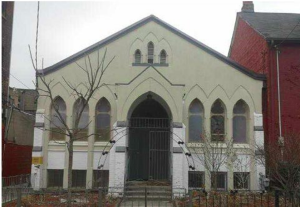
Front (east) elevation (HIA by GBCA, March 2026).
