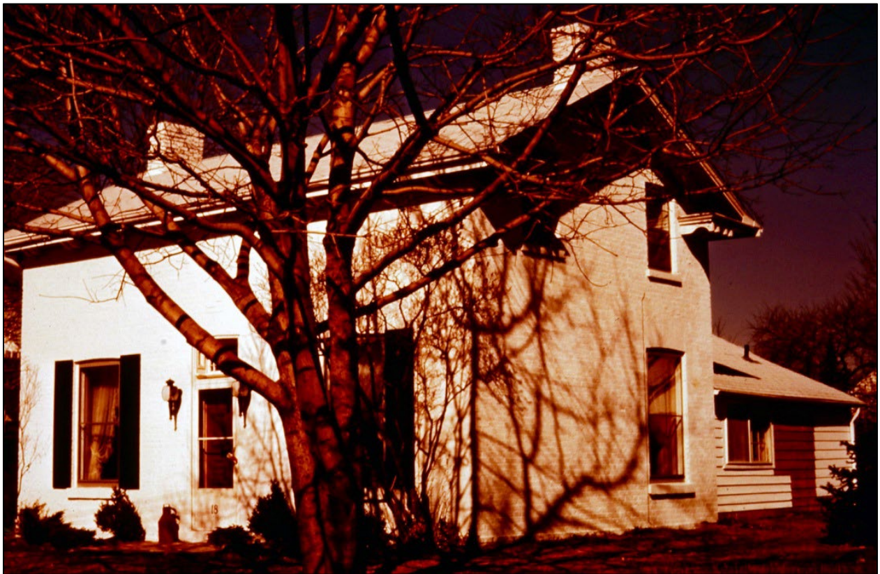
Figure 9: Primary (southeast) facade of 18 Great Oak Drive, c.1966 (Etobicoke Historical Society).
