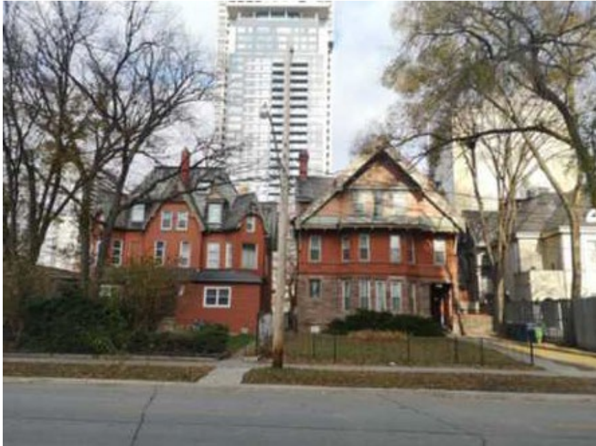
South (principal) elevations of the properties at 164-166 and 168 Isabella Street. (GBCA, 2025)
