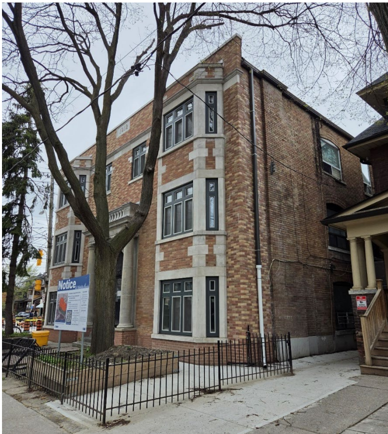
West and south elevations of 1501 Queen Street West, looking northeast (Heritage Planning, 2026).
