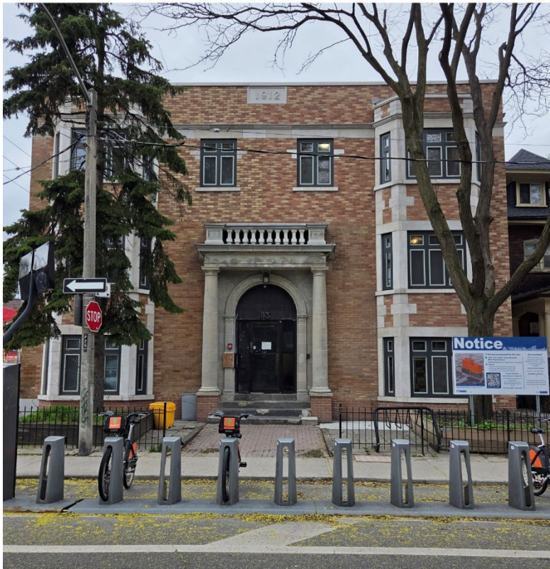
West elevation of 1501 Queen Street West, looking east (Heritage Planning, 2026).
