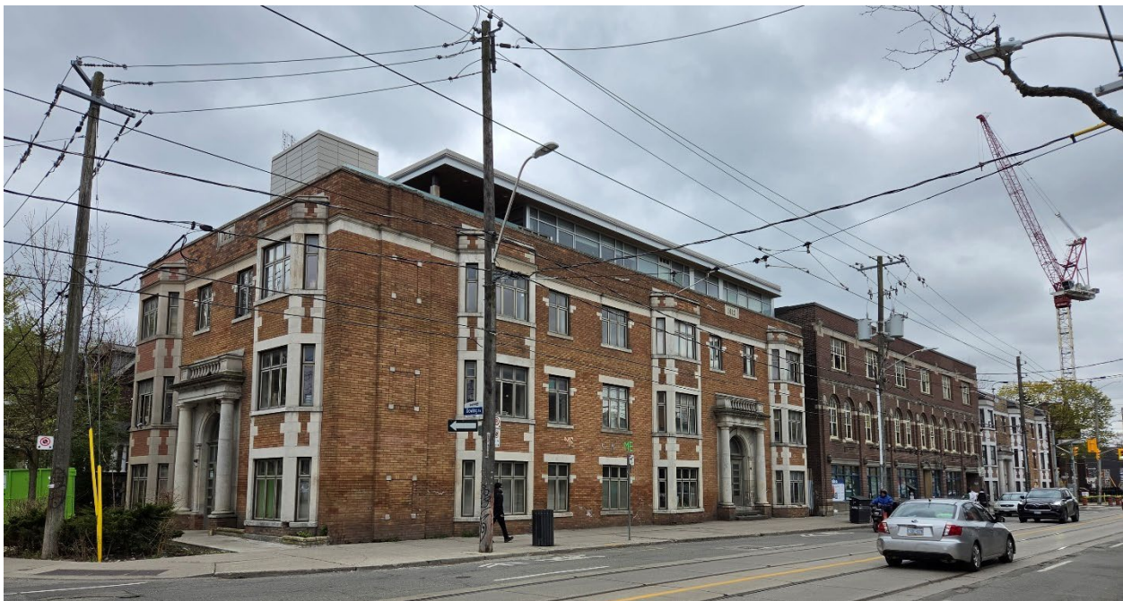
View looking southwest along Queen Street West showing (left to right) 194 Dowling Avenue, 1497 Queen Street West, and 1501 Queen Street West (Heritage Planning, 2026).
