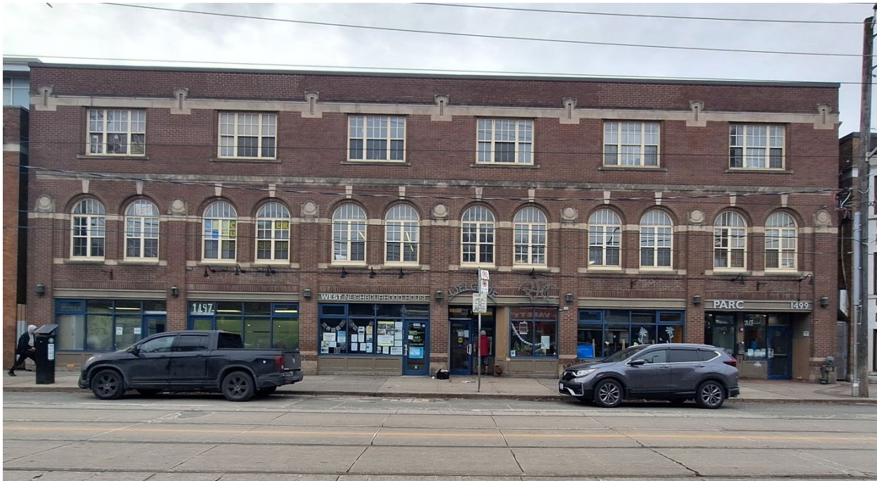
North elevation of 1497 Queen Street West, looking south (Heritage Planning, 2025).
