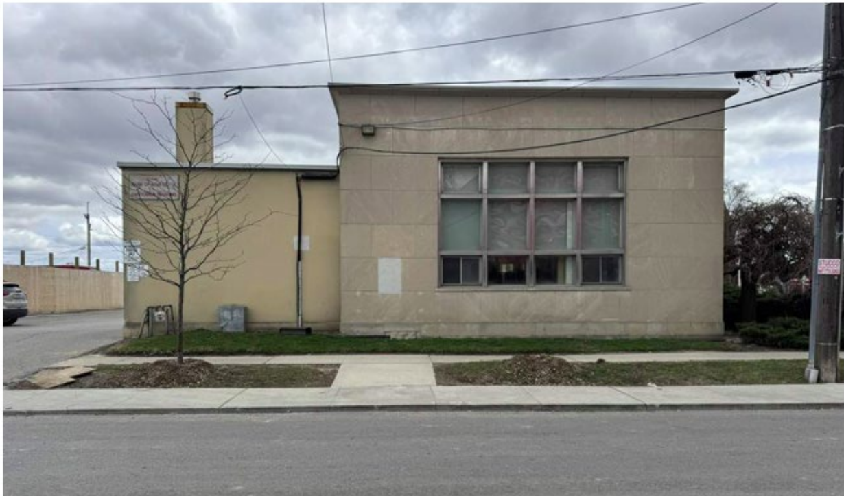
Side elevation of 1151 Weston Road (HIA by Giaimo, March 2026).
