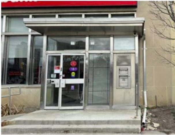
Close-up photograph showing the vestibule on the front elevation (HIA by Giaimo, March 2026).
