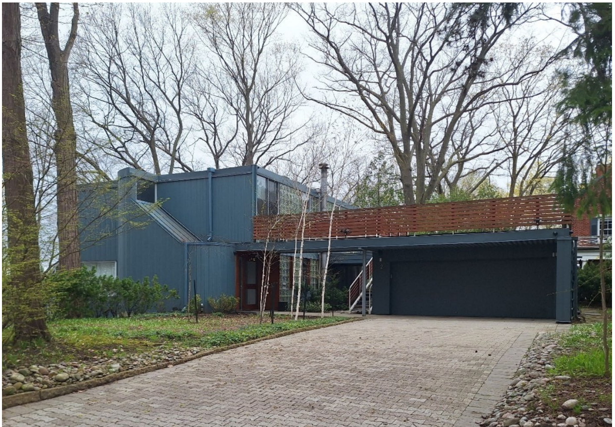
Figure 4 View of the north and east elevation of 2 Hedgewood Road. Note the Stelcolour cladding has been painted and the pipe railings on the garage rooftop patio have been overlaid with wood slats (Heritage Planning, 2026).
