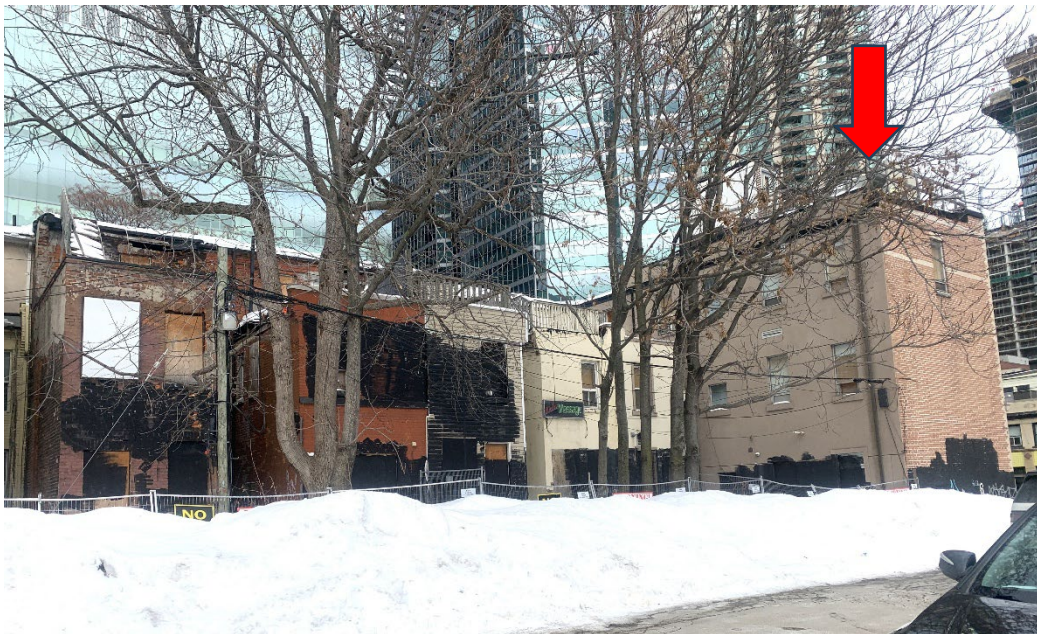
Figure 11: current photograph, looking northeast at the west and south elevations of the subject property. (Heritage Planning, February 2026)
