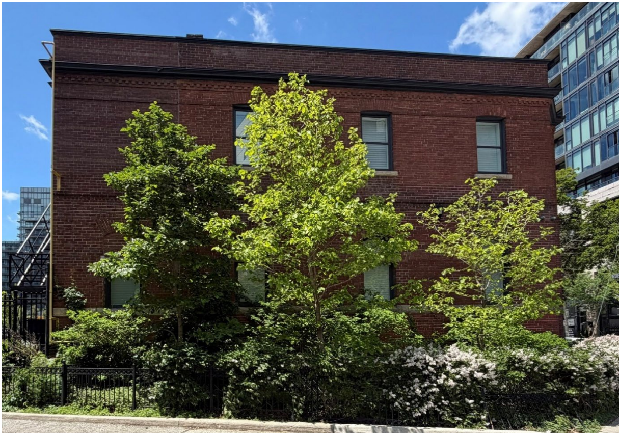
Figure 3: East façade, 2026 (City of Toronto Heritage Planning)
