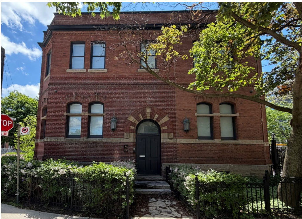
55 Sudbury Street, 2026 (City of Toronto Heritage Planning)
