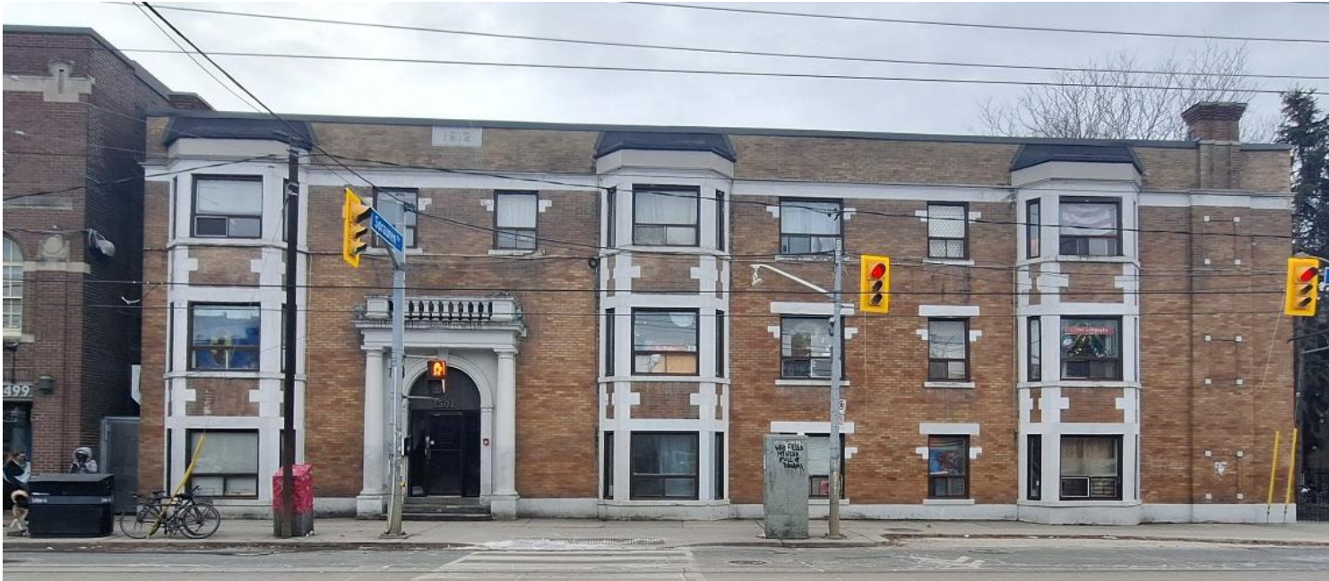
North elevation of 1501 Queen Street West, looking south (Heritage Planning, 2025).
