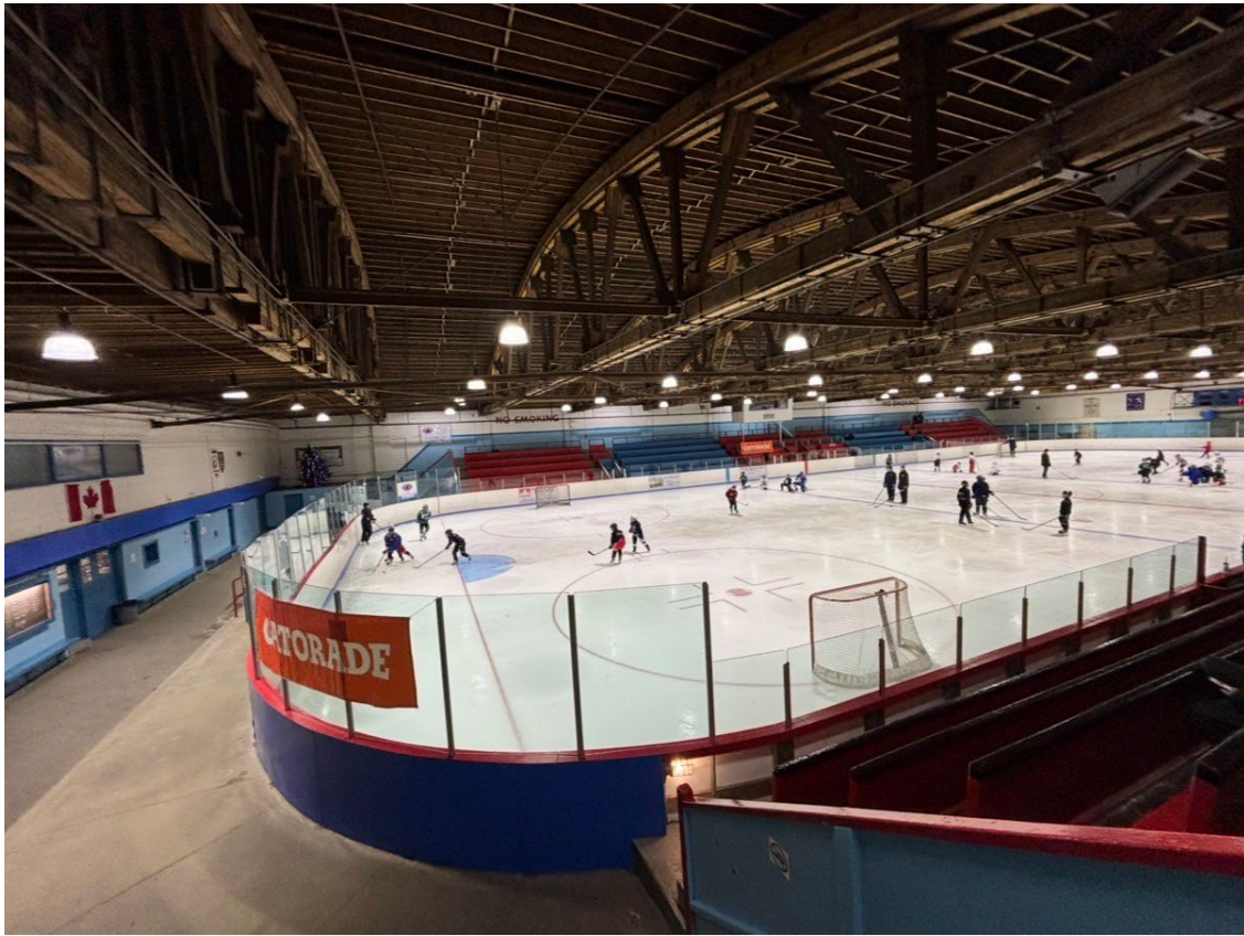
Figure 6: Interior view showing the ice surface and heavy-timber truss roofing system, 2026 (City of Toronto Heritage Planning)
