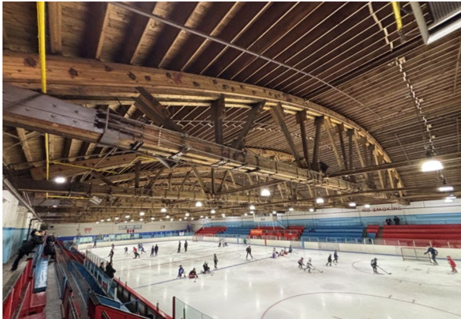
2125 Lawrence Avenue West – interior view (Heritage Planning, 2026)
