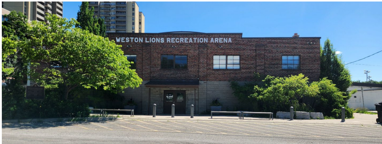
Figure 1: Main (south) façade of the arena, 2026 (City of Toronto Heritage Planning)
