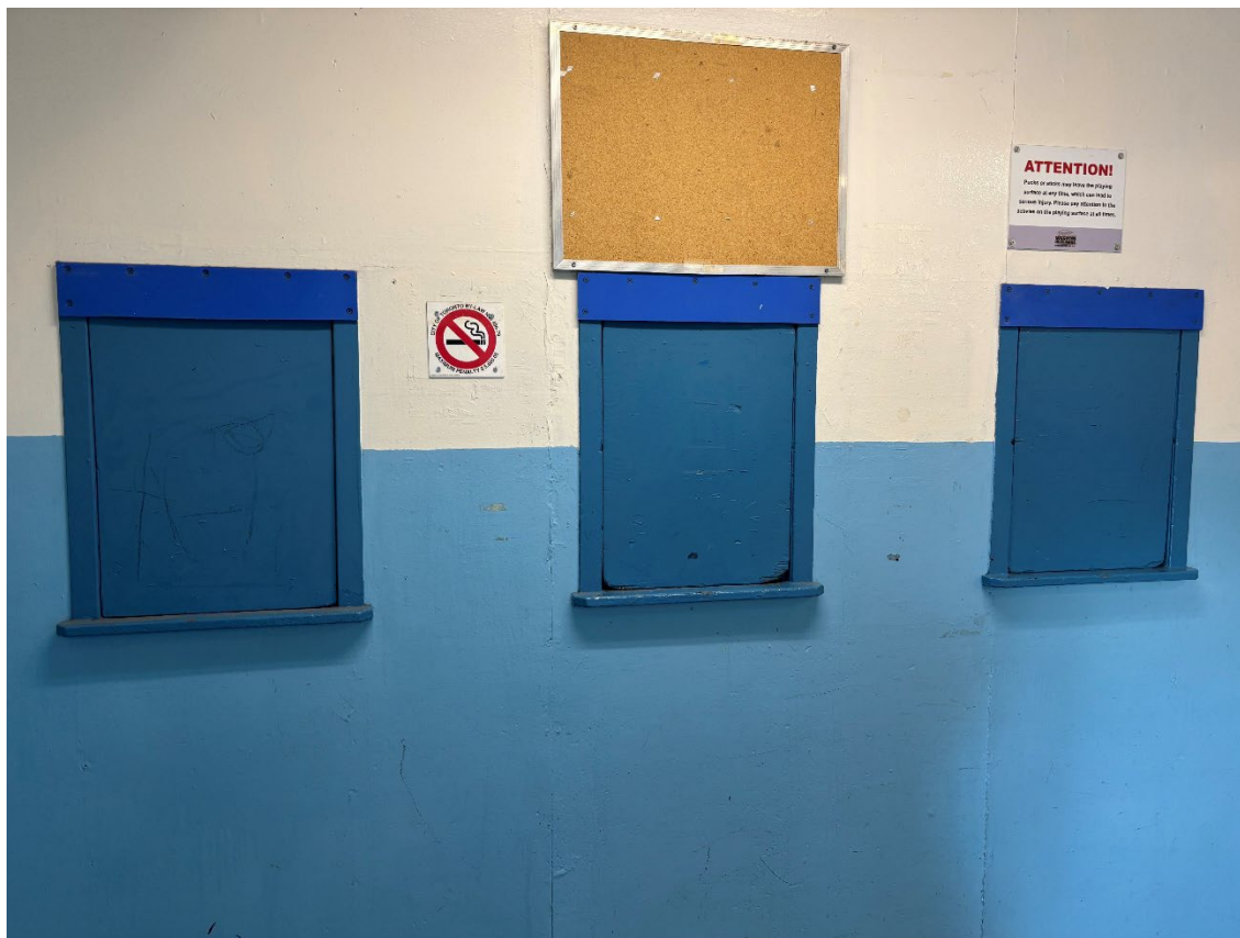
Figure 10: Lobby ticket windows, 2026 (City of Toronto Heritage Planning)
