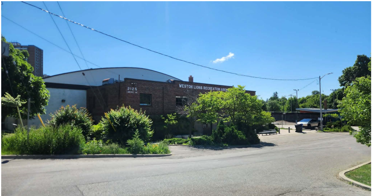
Figure 2: Oblique view of the main (south) façade, 2026 (City of Toronto Heritage Planning)
