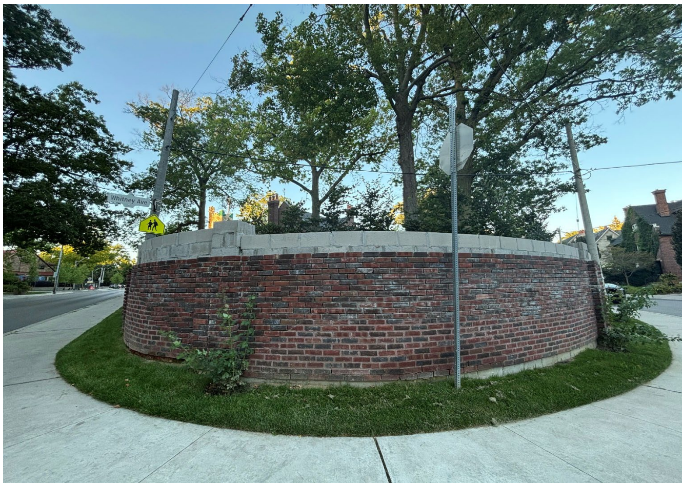
Figure 4: Detailed view of existing wall structure looking northeast towards 2 Whitney Avenue from corner of Glen Road and Whitney Avenue (City of Toronto, August 2025).
