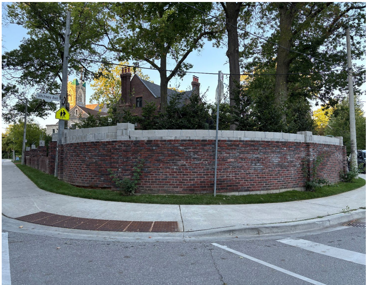
Figure 3: View of existing wall structure looking northeast towards 2 Whitney Avenue from the corner of Glen Road and Whitney Avenue (City of Toronto, August 2025).
