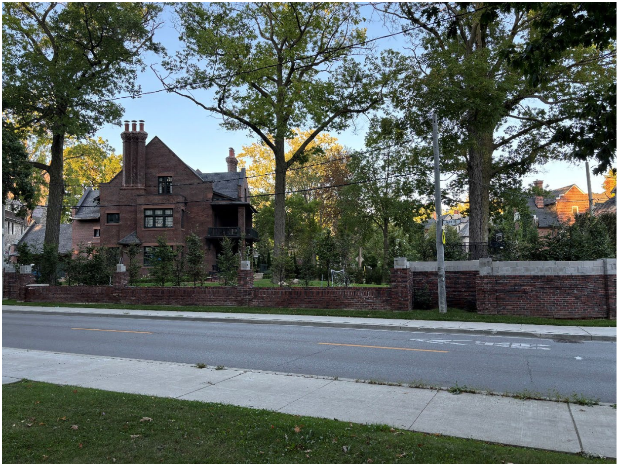
Figure 2: View of existing wall structure looking east toward 2 Whitney Avenue from Glen Road (City of Toronto, August 2025).
