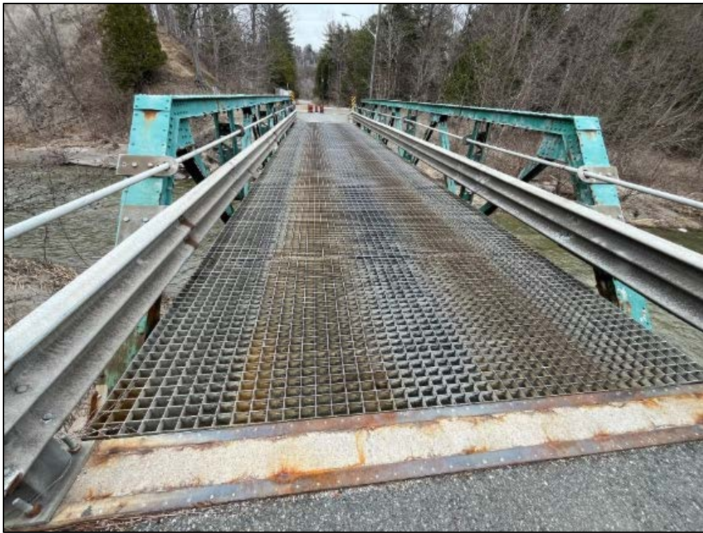
Stotts' Bridge deck, looking west, with expansion joint in the foreground (ASI, 2025)
