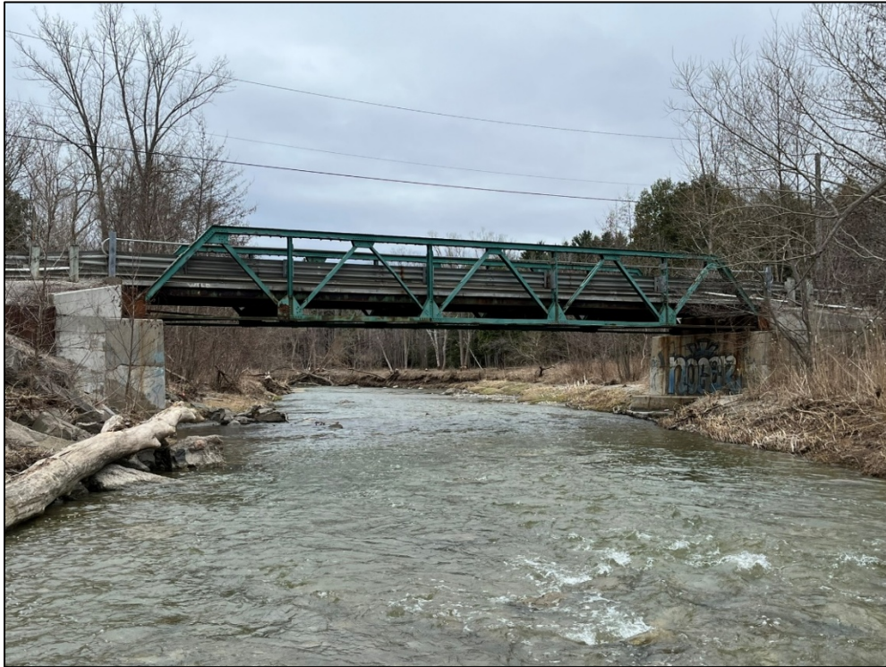
View of the north elevation of Stotts' Bridge, looking south (ASI, 2025)
