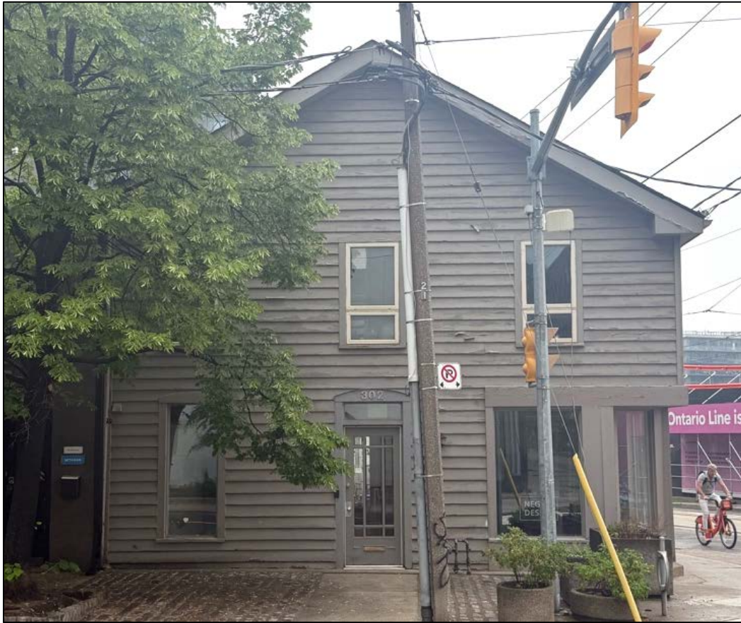
Figure 17: Primary (west) facade of 302 King Street East (June 2026, Alex Corey).
