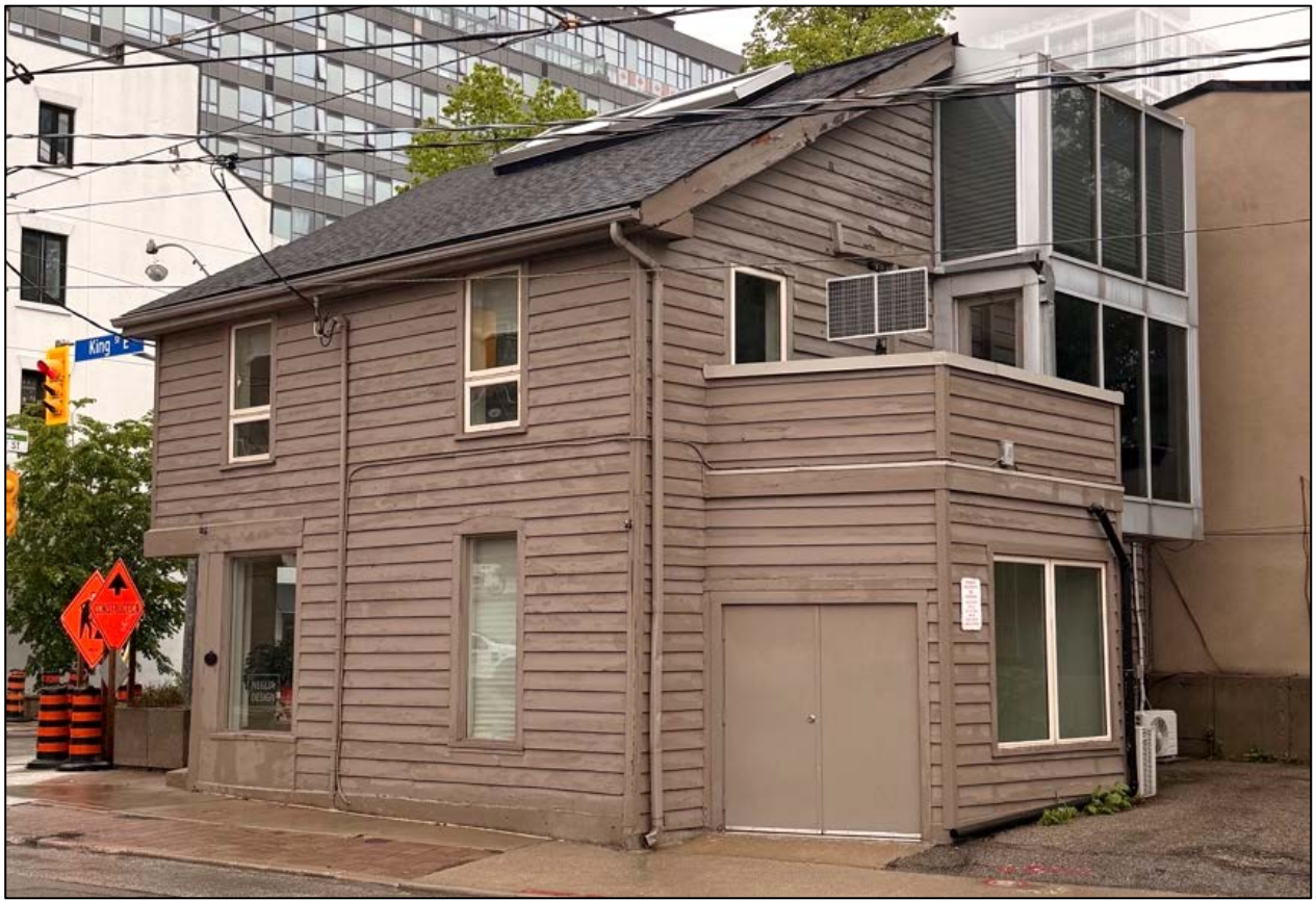
Figure 19: South-east facades of 302 King Street East showing one storey addition with two storey addition behind (May 2026, Alex Corey).
