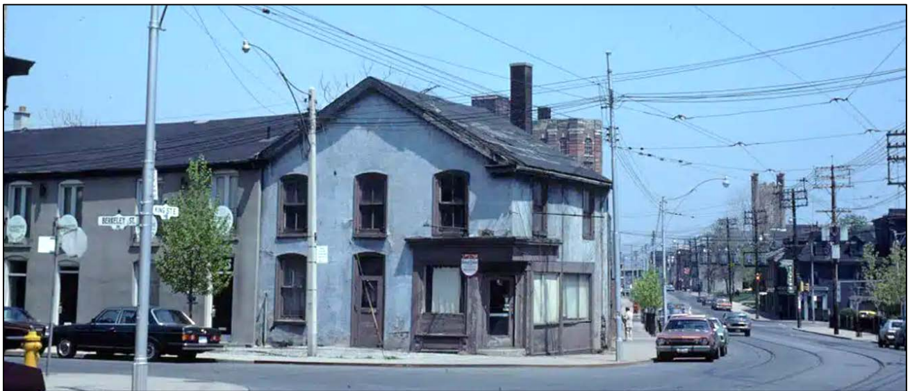
Figure 10: 302 King Street East, prior to 1981 renovations, showing former storefront, windows with casing and stucco cladding, 1979. City of Toronto Archives.
