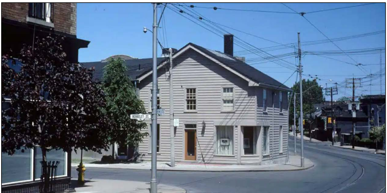
Figure 14: 302 King Street East following renovations, 1981. City of Toronto Archives.
