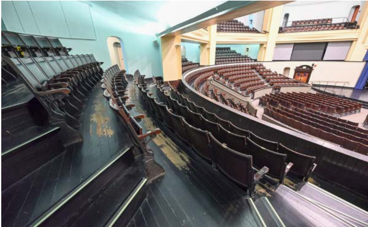
Representative view of the gallery spaces on the second floor (Source: ERA Architects, 2025).
