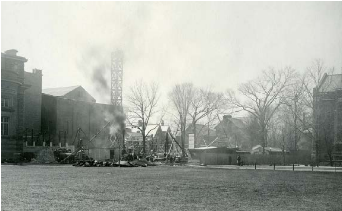
Initial site preparation during the construction of Simcoe Hall (c. April 1923). The northernmost apse of Convocation Hall is visible at far left (Source: University of Toronto Archives).
