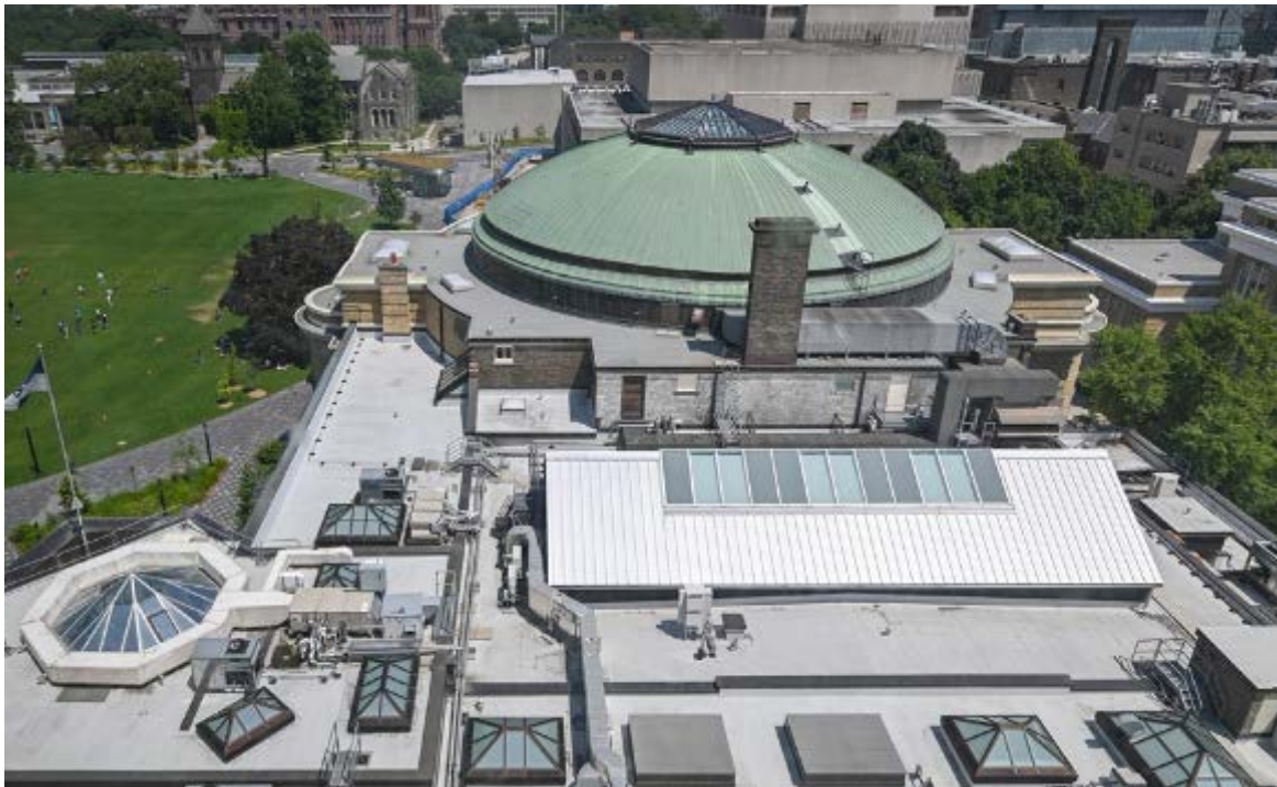
View of the roof of Convocation Hall and Simcoe Hall. The aperture of the multi-purpose assembly hall that was subsumed into Simcoe Hall is visible below the copper dome (Source: ERA Architects, 2025).
