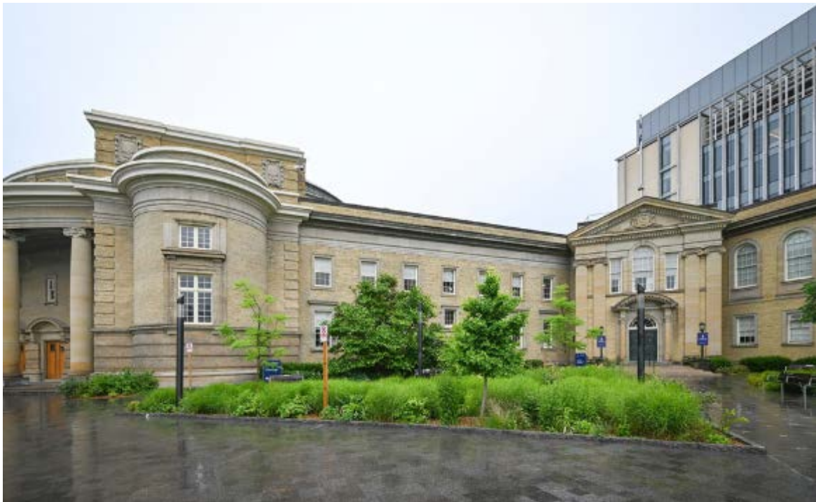
North elevation of infill wing (centre) and northeast elevation of Simcoe Hall (right), showing the relationship with Convocation Hall (left) (Source: ERA Architects, 2025).
