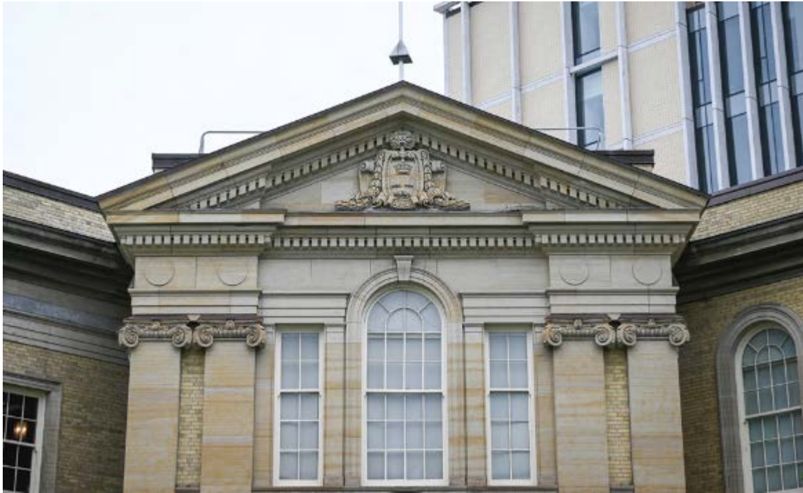
Detail view of masonry carvings on the principal elevation of Simcoe Hall (Source: ERA Architects, 2025).
