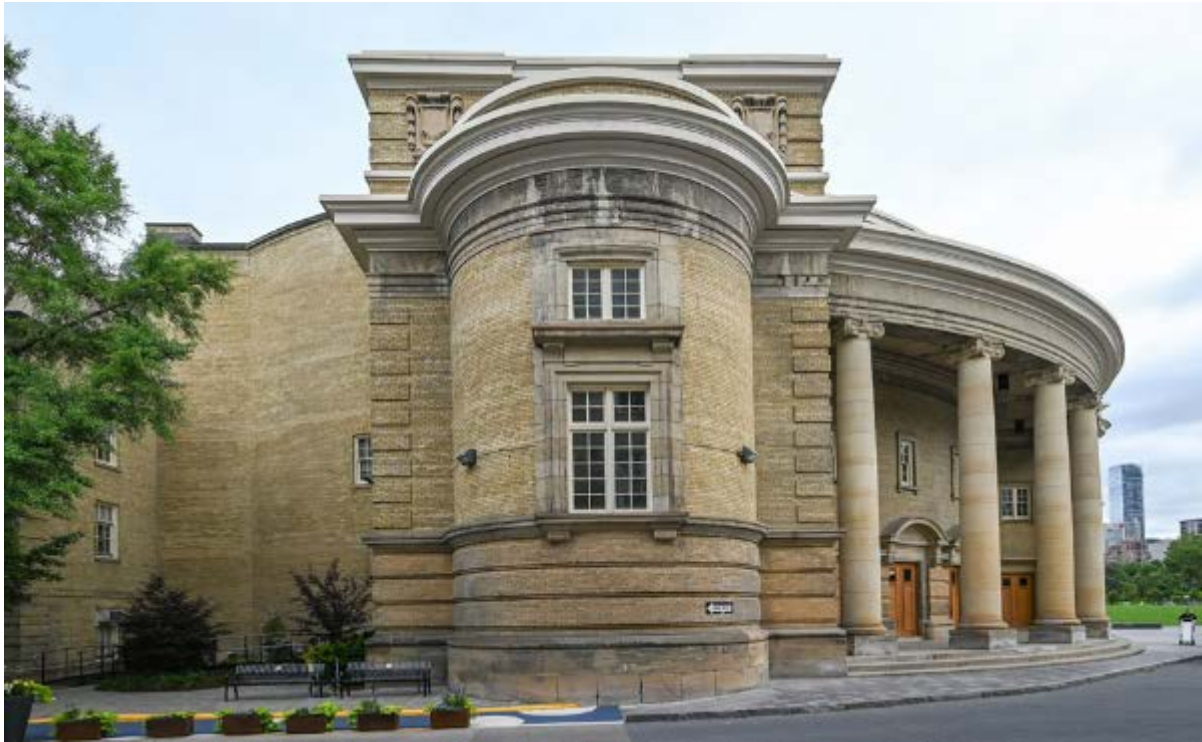
South elevation of Convocation hall showing the southeast loggia and the expanse of buff brick of the southwest elevation (Source: ERA Architects, 2025).
