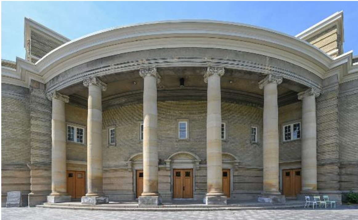
Northeast loggia of Convocation Hall (Source: ERA Architects, 2025).
