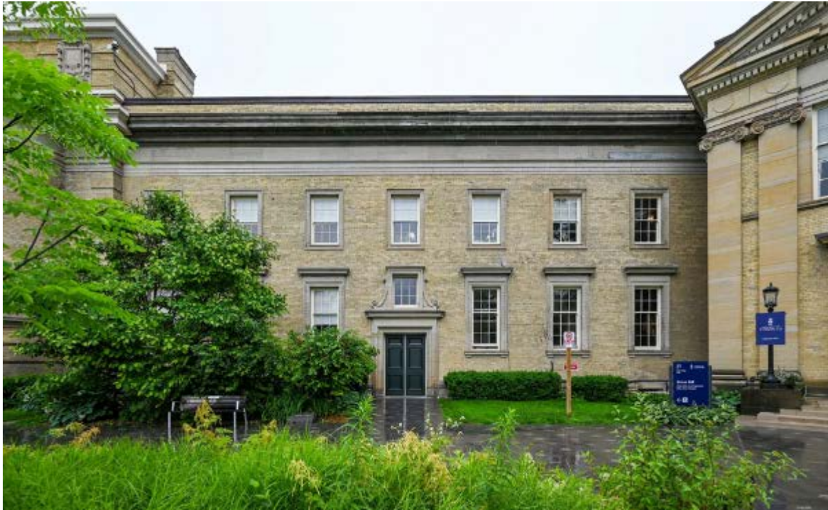
North elevation of the Simcoe Hall infill wing (Source: ERA Architects, 2025).
