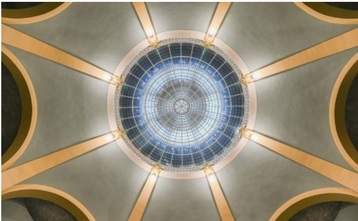
Detail of interior domed ceiling and coloured-glass laylight (Source: ERA Architects, 2025).
