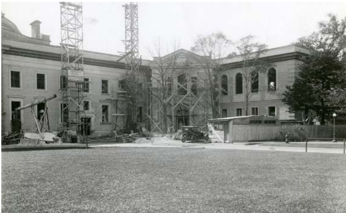
Northeast elevation, including primary entrance, during construction in October 1923 (Source: University of Toronto Archives).
