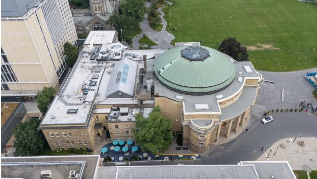
The south elevations of Simcoe Hall and Convocation Hall (City of Toronto, 2025)
