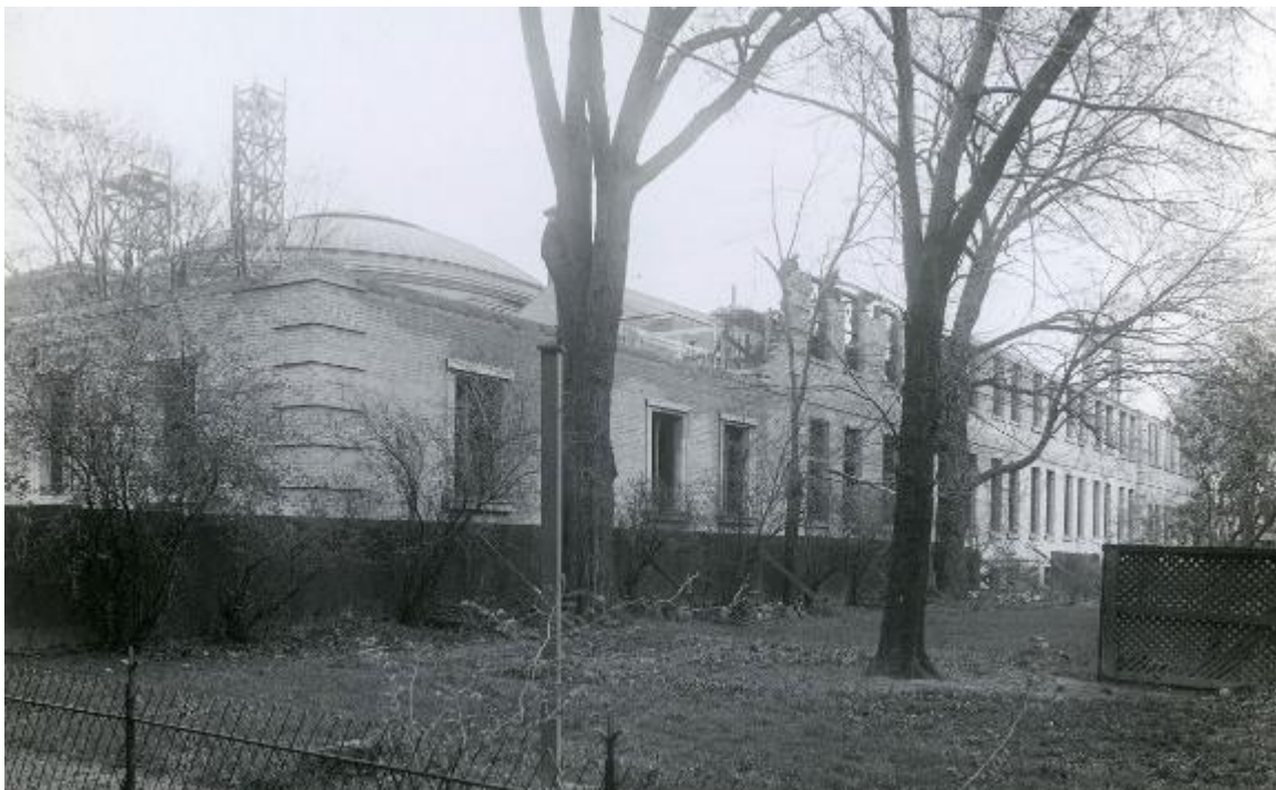
View of the west elevation of Simcoe Hall under construction in May 1923 (Source: University of Toronto Archives).
