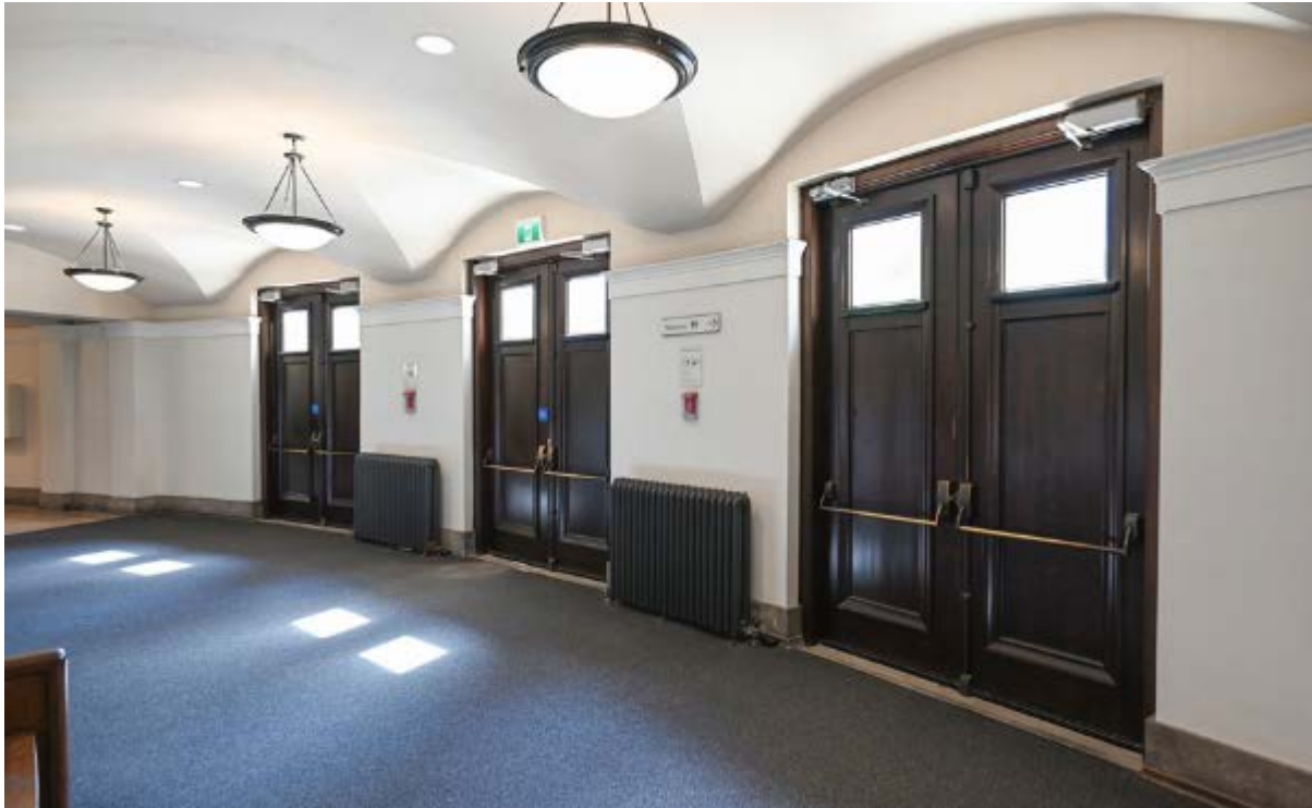
View of one of two sets of three double doors leading to the loggias (Source: ERA Architects, 2025).
