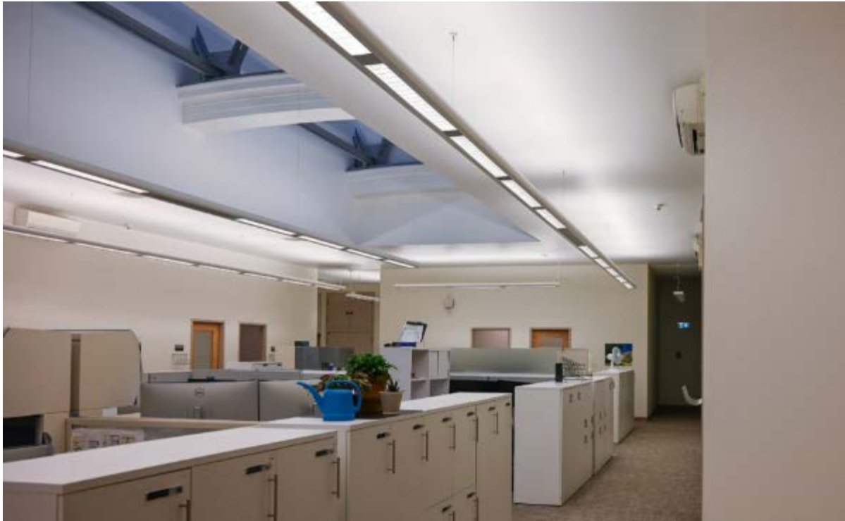
Representative office space on the second floor of Simcoe Hall. The skylight aperture and arched ribs are remnants of a 1909 utilitarian addition to Convocation Hall (Source: ERA Architects, 2025).
