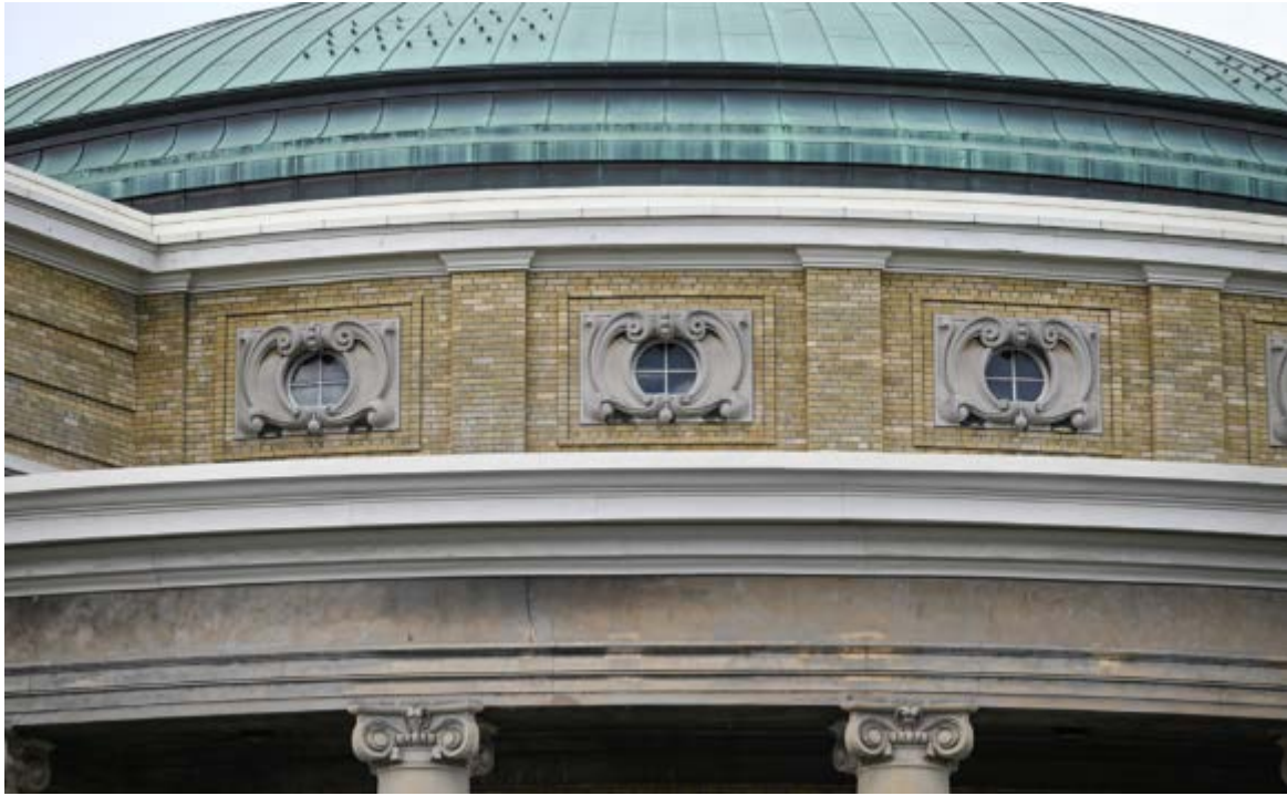
Detail of the entablature, roundel windows with carved stone surrounds, and copper dome on the northeast elevation (Source: ERA Architects, 2025).
