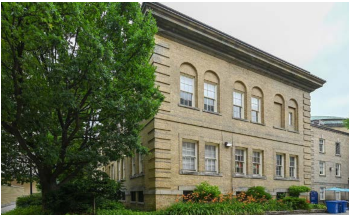
South elevation of Simcoe Hall as it fronts Galbraith Road (Source: ERA Architects, 2025).
