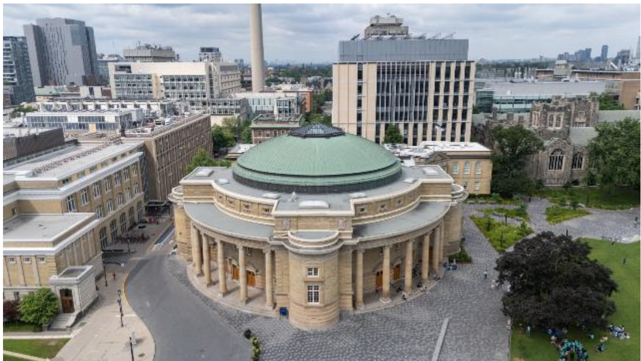
East elevation of Convocation Hall, showing both loggias. Simcoe Hall is visible to the rear of Convocation Hall (City of Toronto, 2025)
