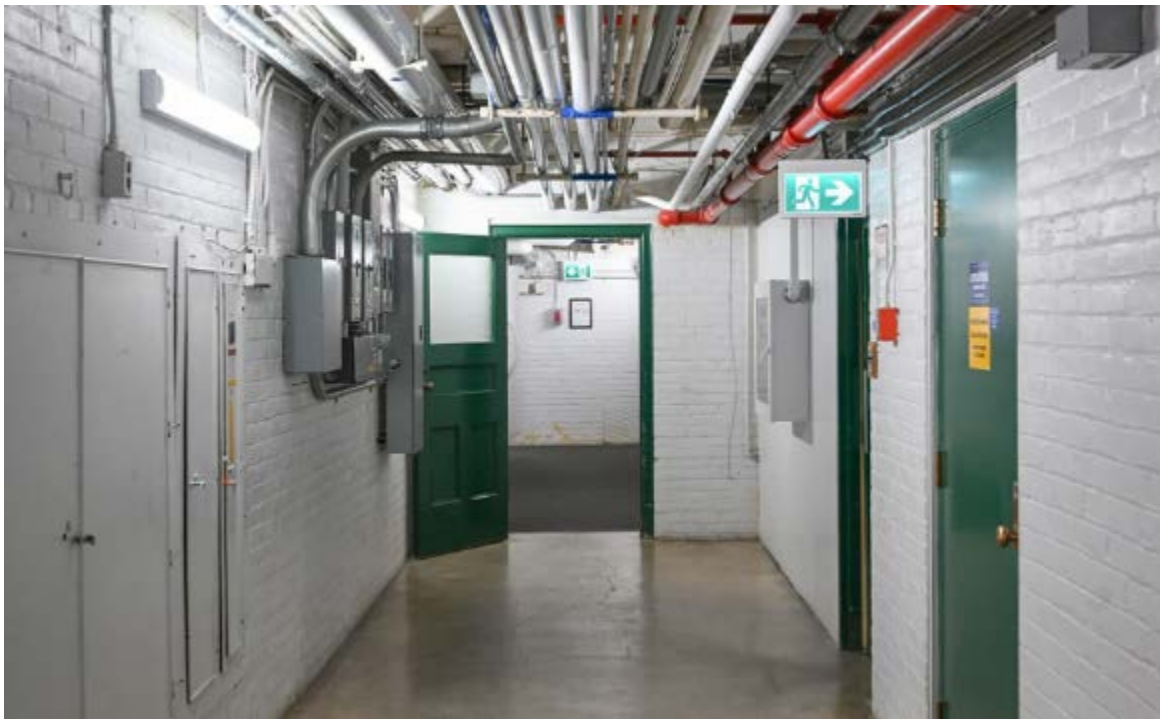
Representative basement corridor space (Source: ERA Architects, 2025).
