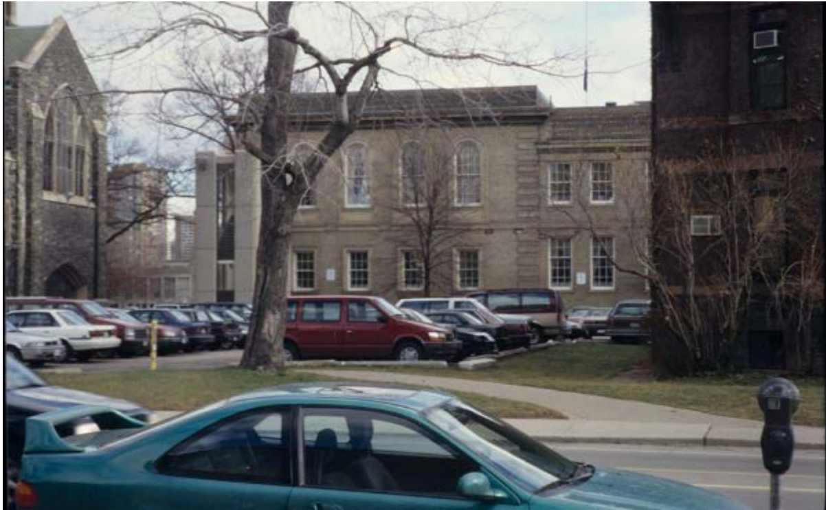
View of the west elevation of Simcoe Hall prior to the construction of the Myhal Centre and the replacement of the 1972 two-storey egress structure with an elevated bridgeway linking Simcoe Hall with the Myhal Centre. Photographed c. 1990 (Source: University of Toronto Archives).
