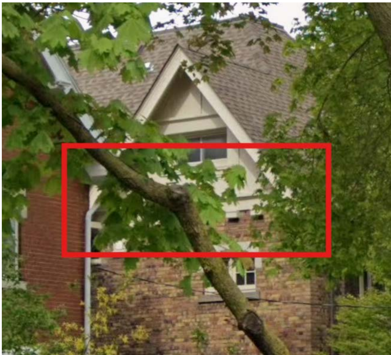
Photo of the east elevation of the existing building at 87 Highland Avenue showing architectural elements found on the east gable, prior to the unauthorized alterations (Google Maps, 2019)
