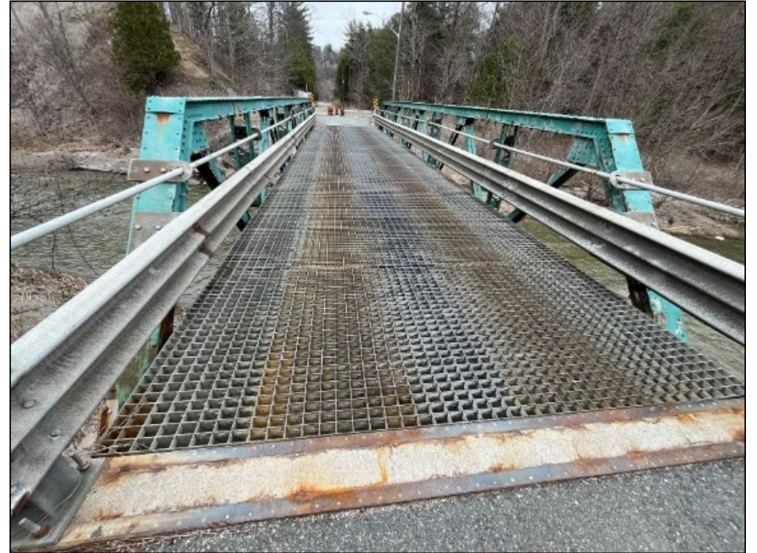
Stotts' Bridge deck, looking west, with expansion joint in the foreground
