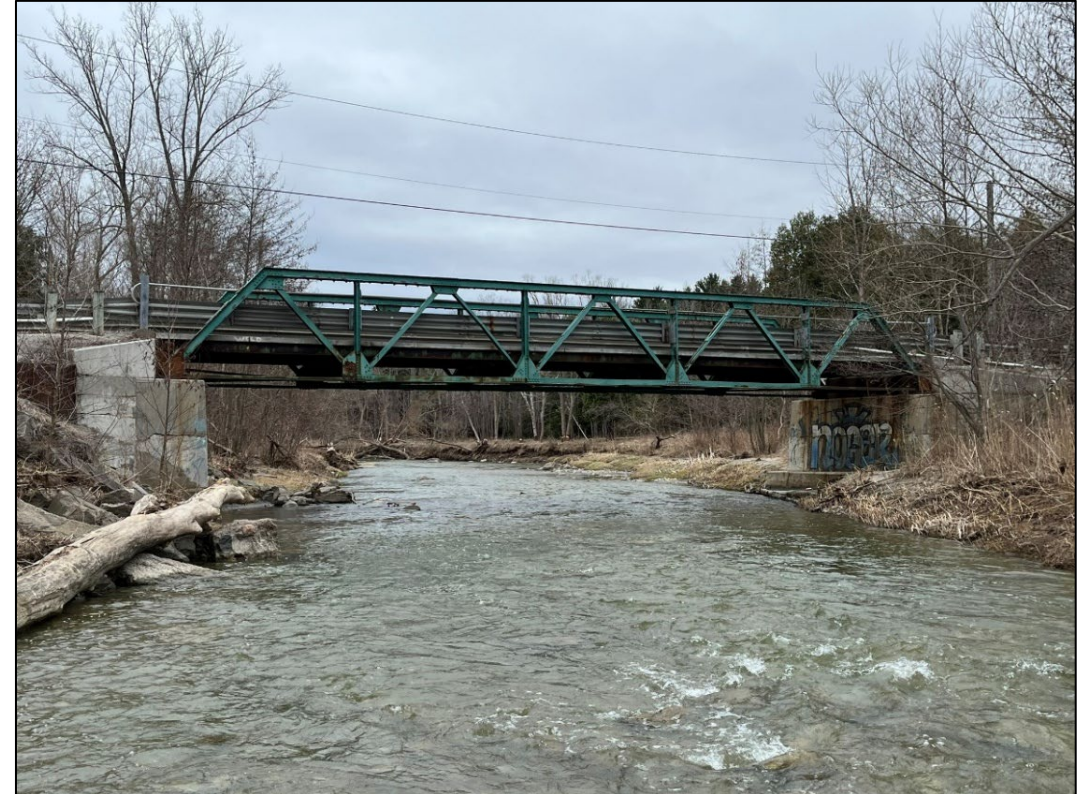
View of the north elevation of Stotts' Bridge, looking south
