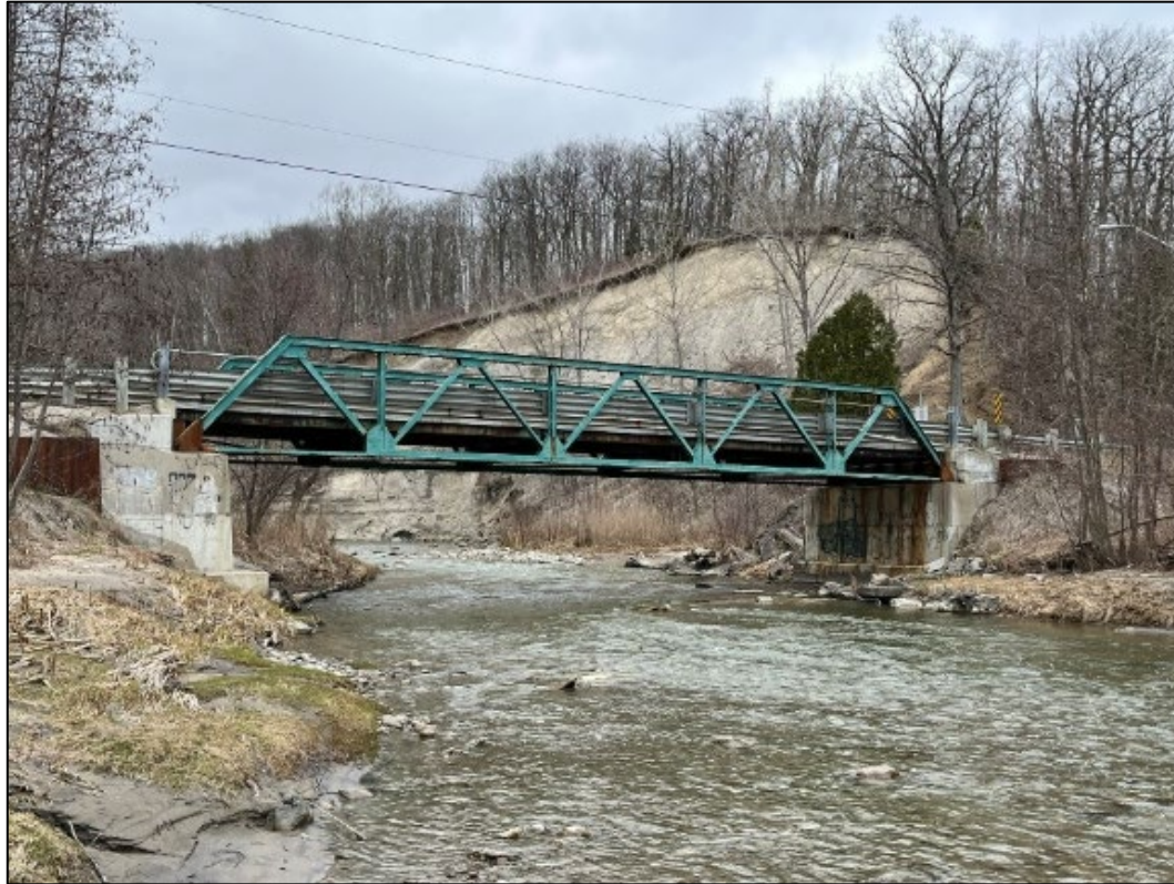
View of the south elevation of Stotts' Bridge, looking northeast
