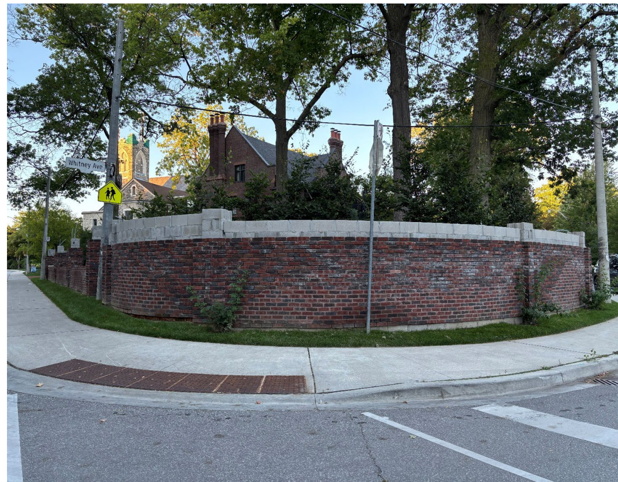
View of wall structure looking south towards 2 Whitney Avenue from Whitney Avenue (City of Toronto, August 2025)
