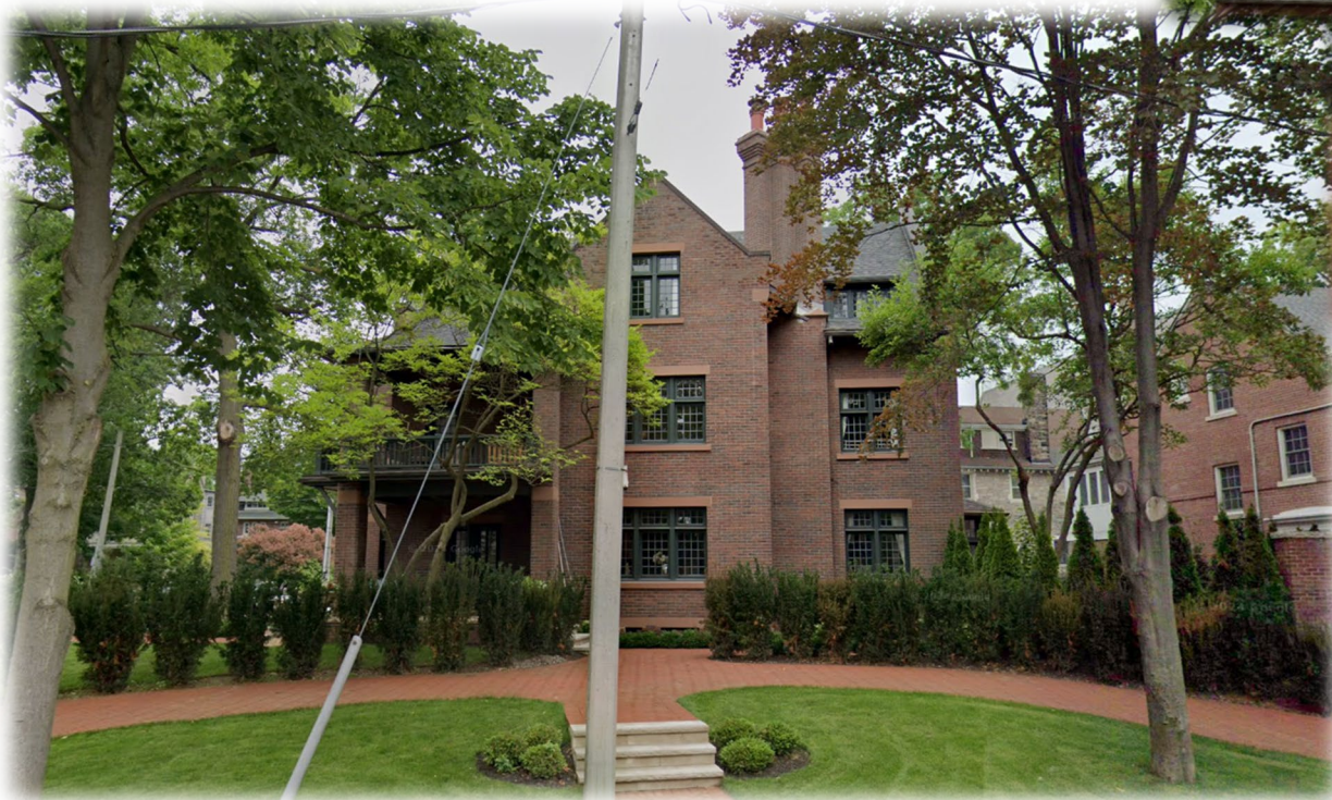
View of south elevation at 2 Whitney Avenue (Google Maps, 2024)
