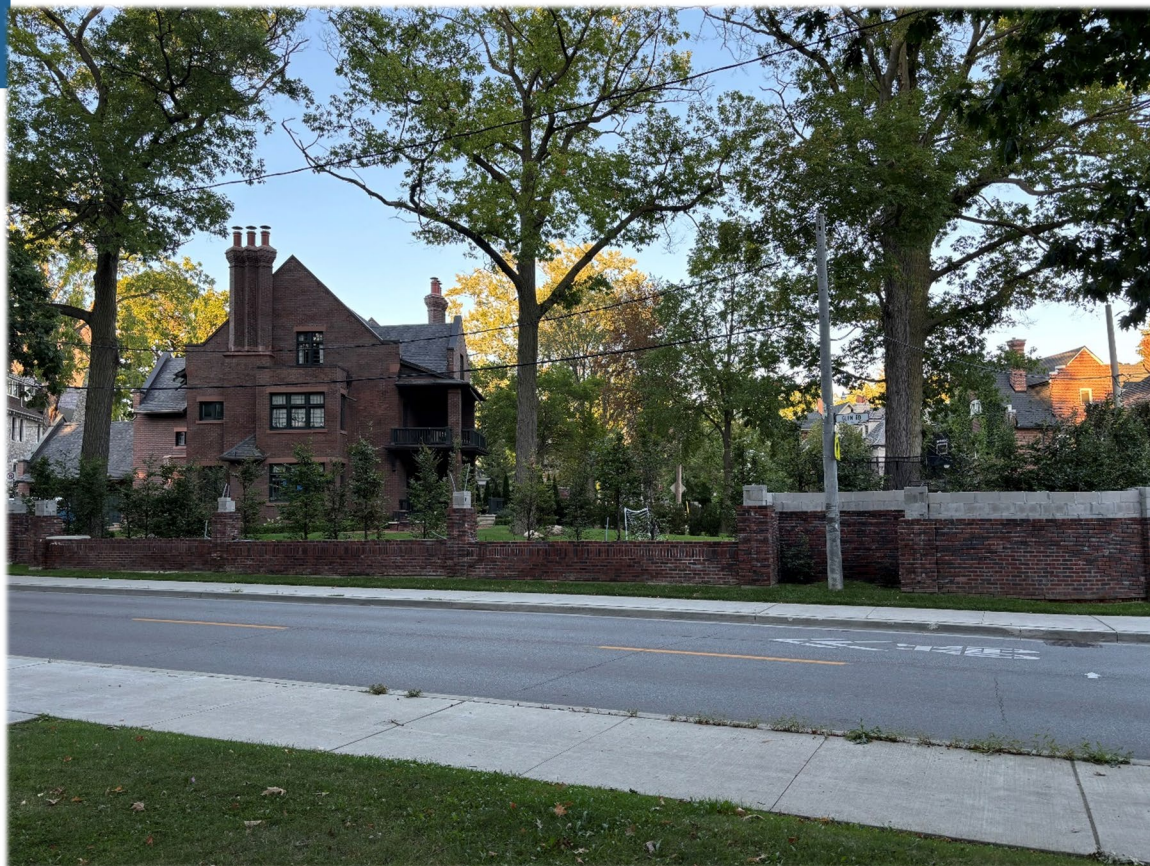
View of wall structure looking east toward 2 Whitney Avenue from Glen Road (City of Toronto, August 2025)
