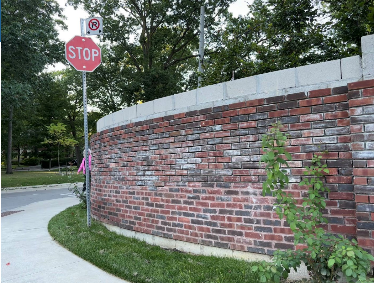
Detailed view of existing wall structure looking west towards Glen Road from corner of Glen Road and Whitney Avenue (City of Toronto, August 2025)
