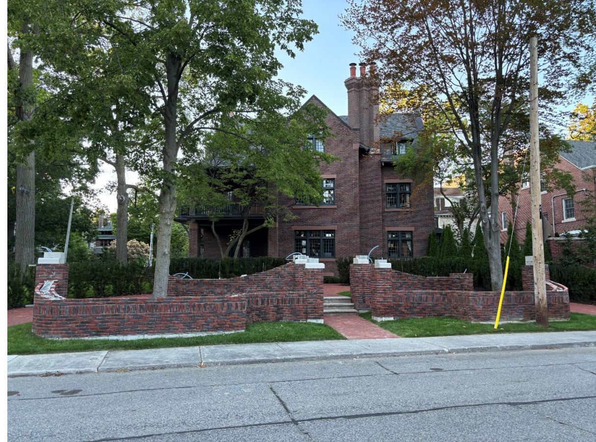
View of existing wall structure looking south towards 2 Whitney Avenue from Whitney Avenue (City of Toronto, August 2025)
