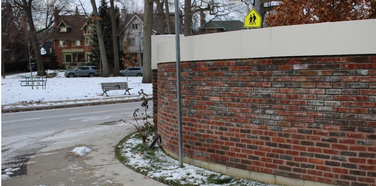
Figure 4: Site exam photo, of the minimal clearance (18 cm) between the stop sign post and the wall.
