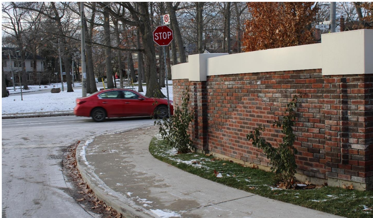
Figure 2: Site exam photo, looking west on Whitney Ave. toward the intersection, taken 25 m back from the intersection of the westbound lane and the southbound lane. The incident brick wall completely blocks the view of southbound traffic from this location.
