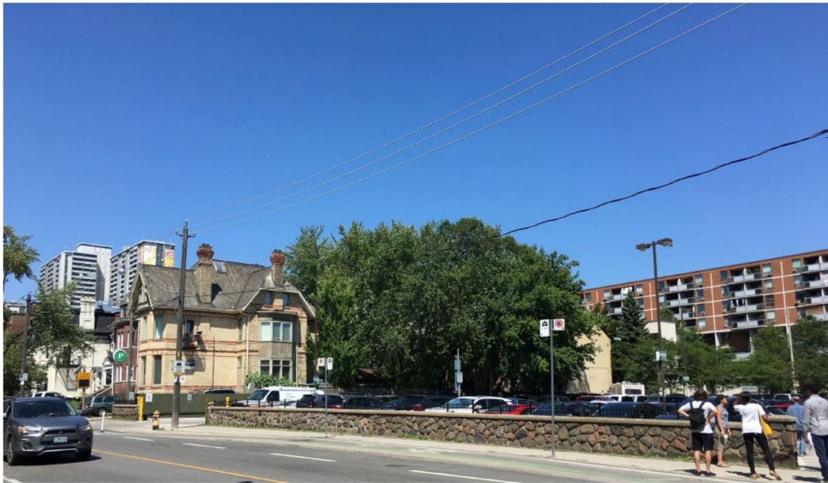
Figure 2. 405 Sherbourne Street looking northeast (ERA Architects Inc., 2020).
