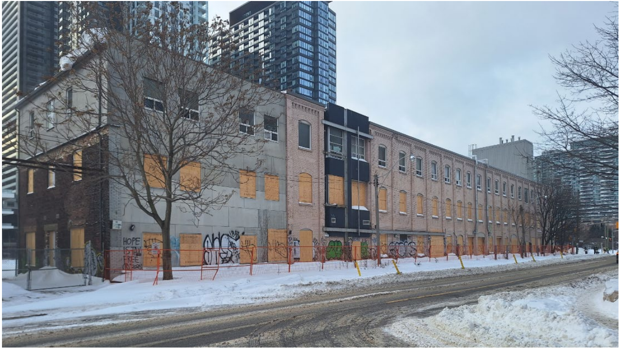
Figure 11 View of Strachan House looking southwest along Wellington Street West showing principal (north) and west elevations (Heritage Planning, 2026).
