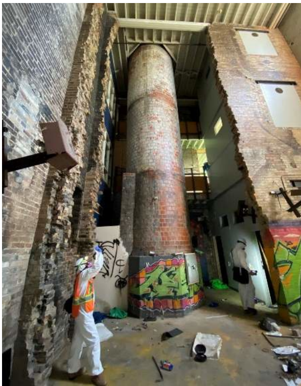
Figure 18 Current interior photo of the 'Town Square' with smokestack (RDH Building Science, 2025).
