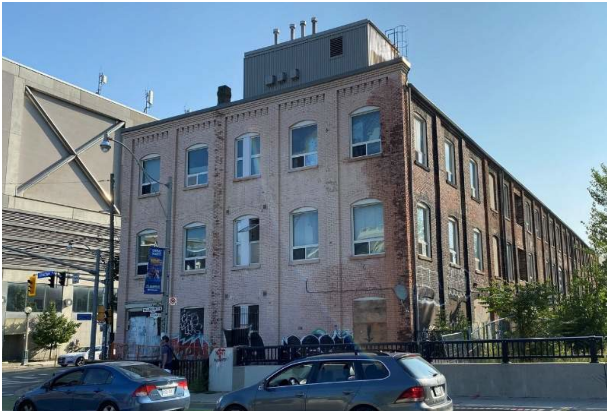
Figure 14 View looking northeast showing the principal (west) and south elevations of Strachan House (RDH Building Science, 2025).
