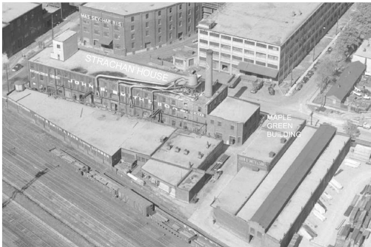
Figure 2 1949 aerial image showing Strachan House with 2 storey east annex, Maple Green Building with lumber sheds, and other outbuildings. Note the prominent 'John B. Smith & Sons' and other painted signage (Ontario Archives).
