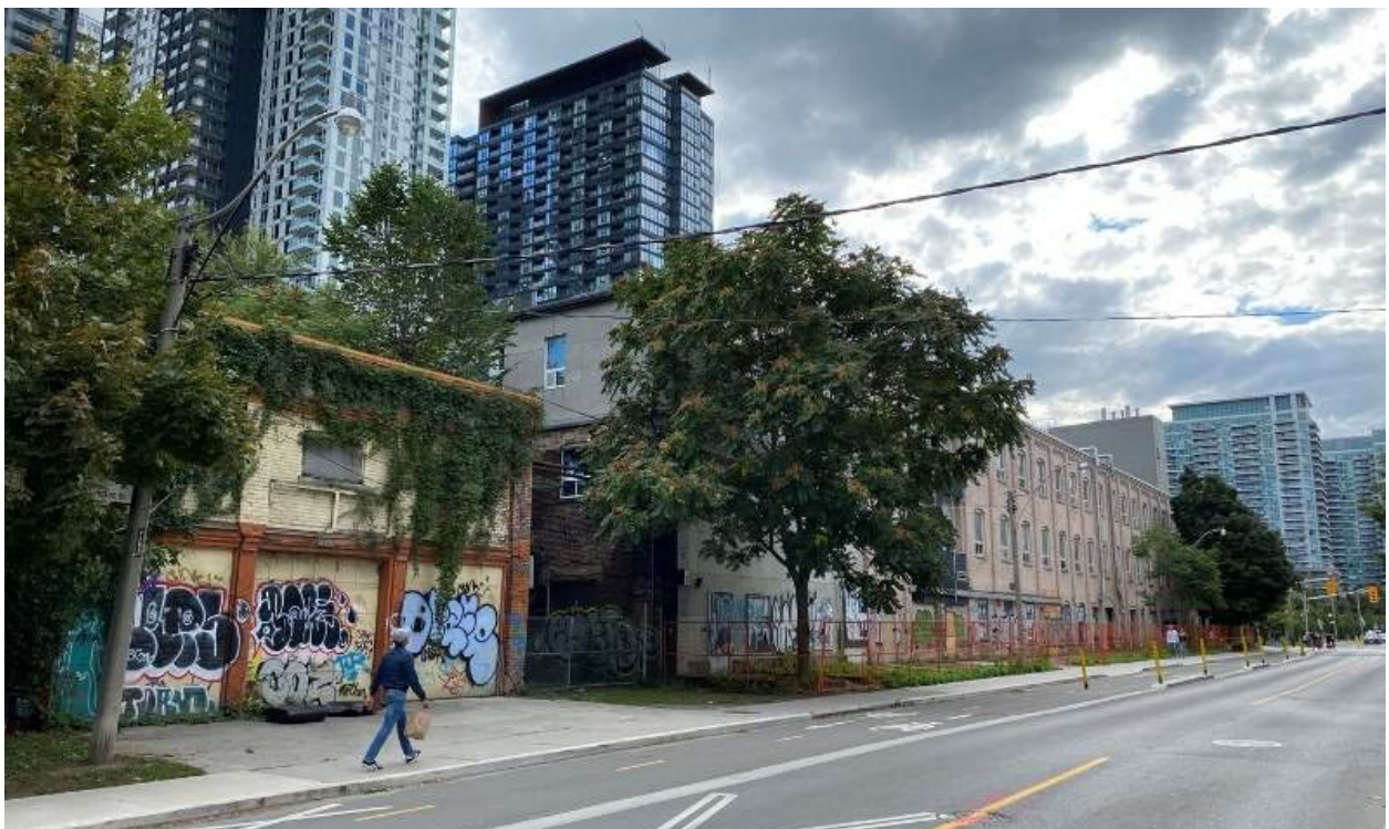
Figure 12 View looking southwest showing north elevations of the Maple Green Building and Strachan House (RDH Building Science, 2025).
