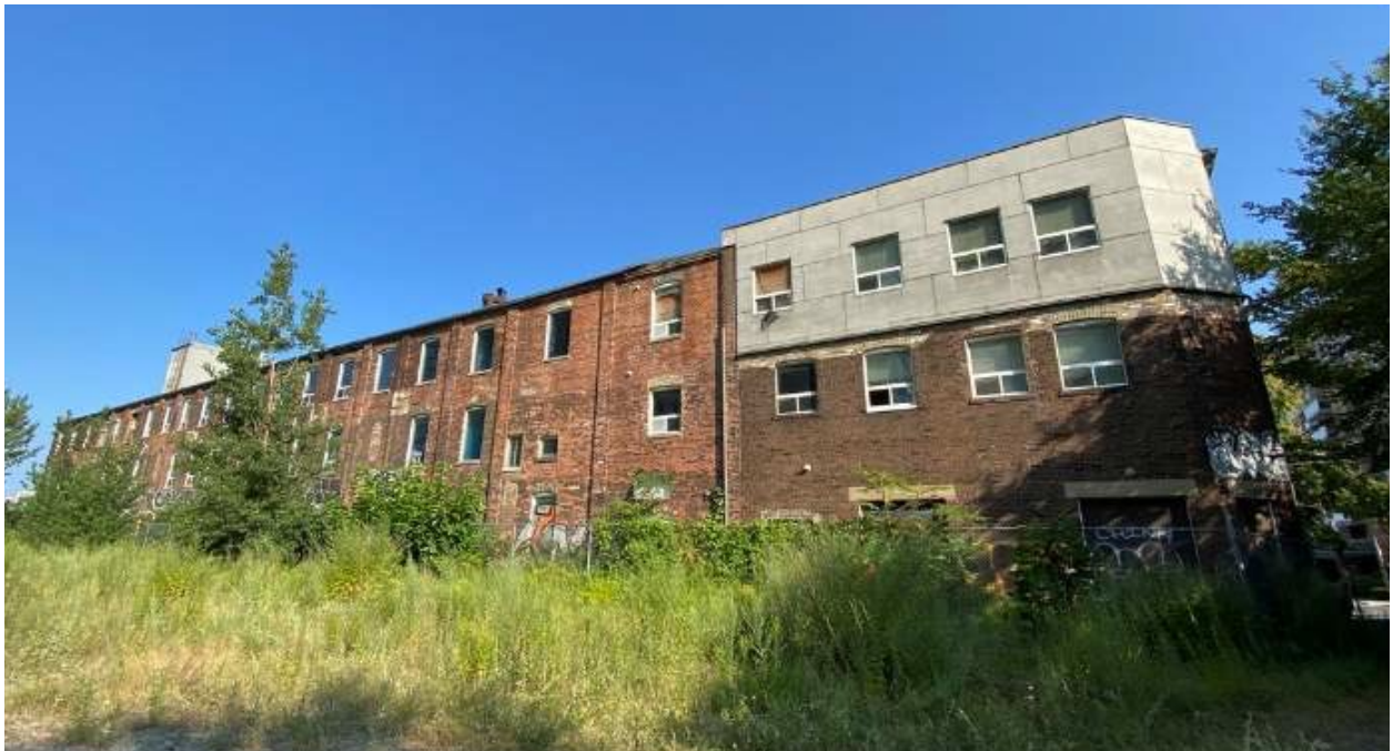
Figure 13 View looking north showing the south elevation of Strachan House (RDH Building Science, 2025).
