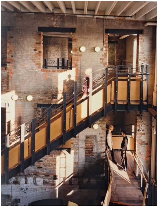
Figure 15 1996 interior photo of Strachan House's three storey atrium known as the 'Town Square' (Toronto Archives).
