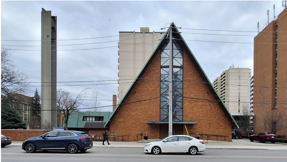
Figure 1 Image of St. Peter's Estonian Evangelical Lutheran Church from Mount Pleasant Road showing (right to left) the Church Building, Auxiliary Wing, and Bell Tower, and columbarium wall (Heritage Planning, 2025).
