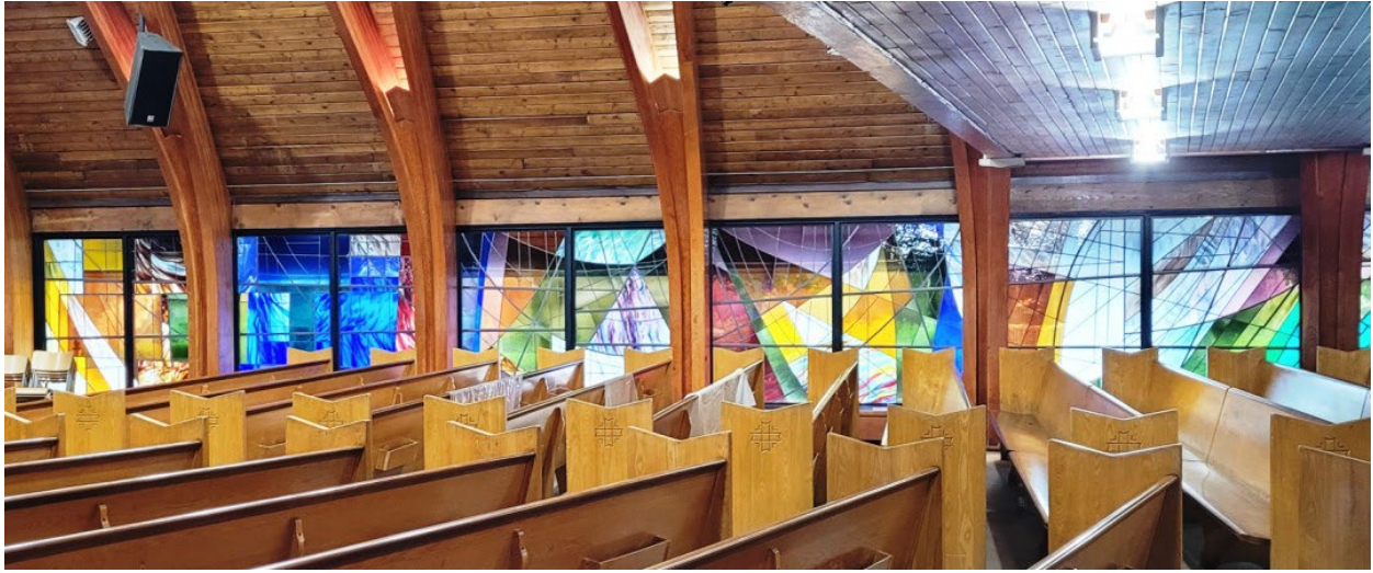
Figure 12 Interior view of south elevation showing coloured glass windows, glulam truss beams and pews (St. Peter's EELC, 2026).
