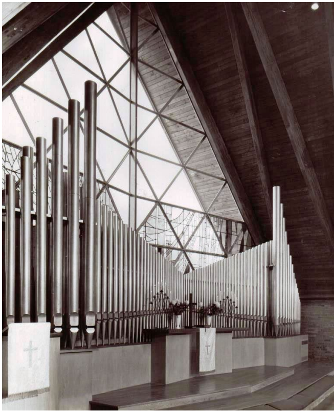
Figure 9 1960s image showing the original altar and east elevation with partially finished coloured glass windows and Pipe Organ (St. Peter's EELC).
