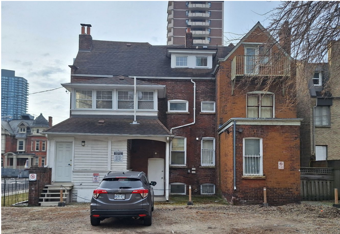
Figure 16 Rear (north) elevation of 122 and 124 Isabella Street (Heritage Planning, 2026).
