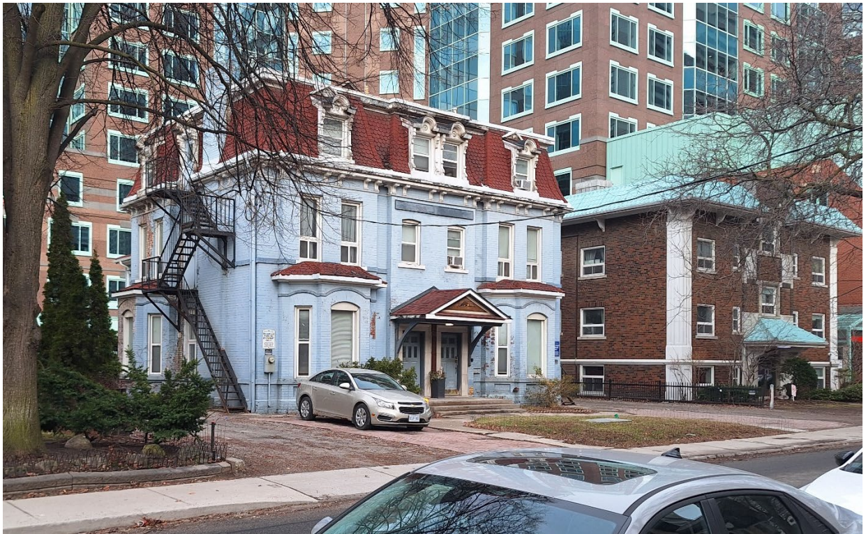
Figure 7 View looking northwest towards south elevation of 38 Huntley Street and principal (east) elevation of 38 and 40 Huntley Street (Heritage Planning, 2026).
