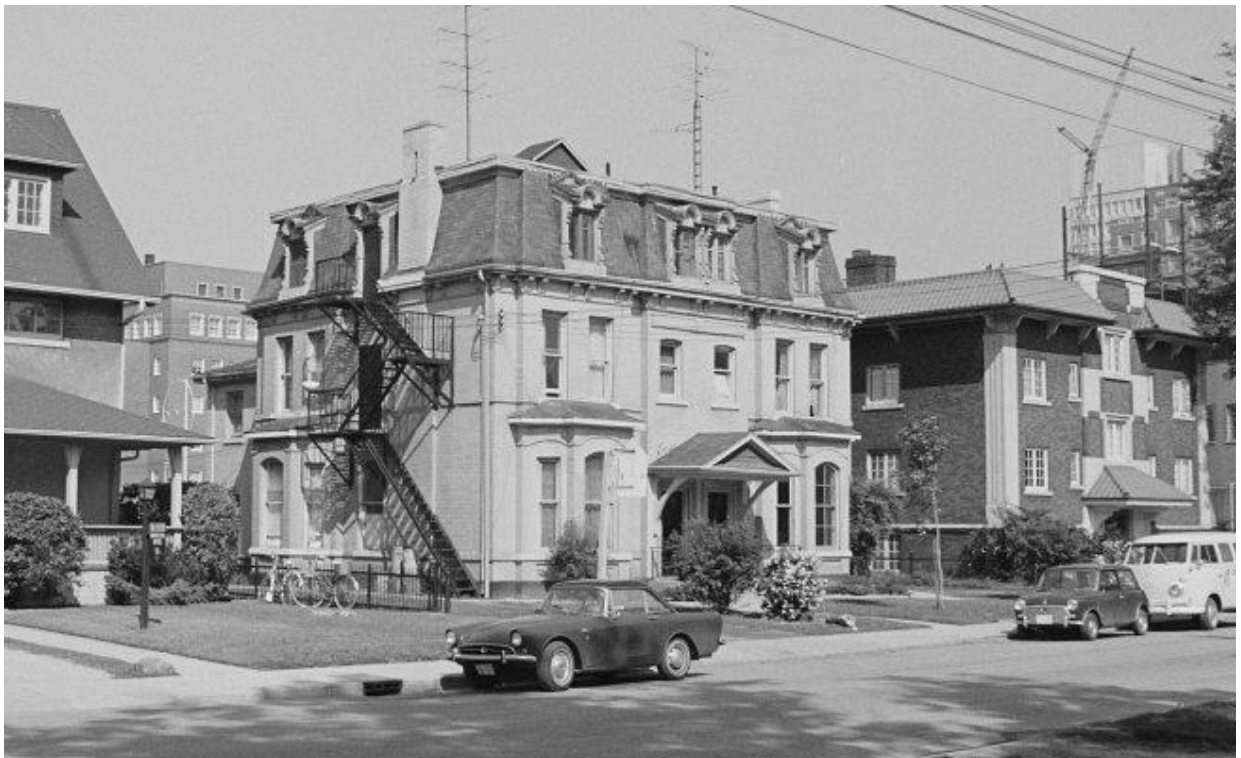
Figure 6 1972 image looking northwest towards south elevation of 38 Huntley Street and principal (east) elevation of 38 and 40 Huntley Street (Toronto Archives).
