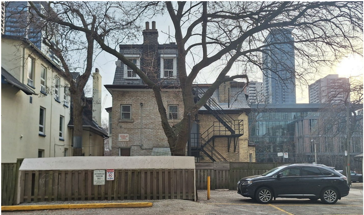
Figure 5 West (rear) elevation of 30 and 32 Huntley Street (Heritage Planning, 2026).
