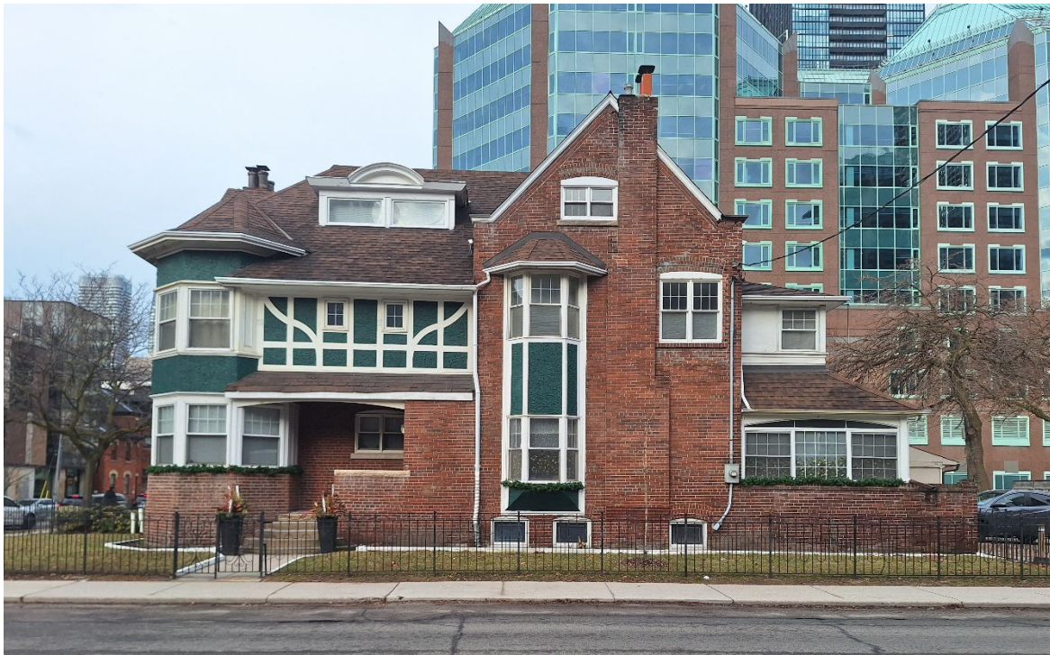
Figure 15 East elevation of 124 Isabella Street (Heritage Planning, 2026).
