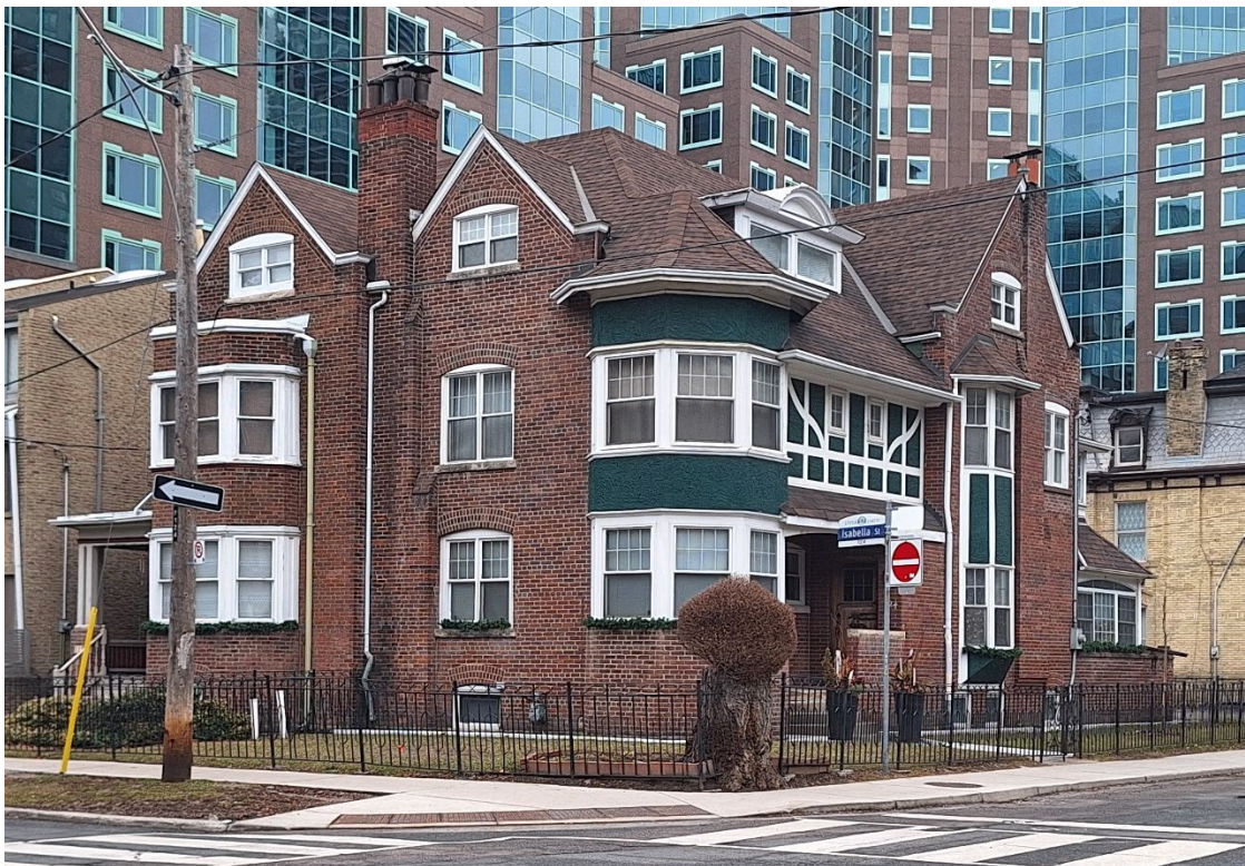
Figure 12 View looking northwest towards the principal (south) elevation of 122 and 124 Isabella Street and east elevation of 124 Isabella Street (Heritage planning, 2026).
