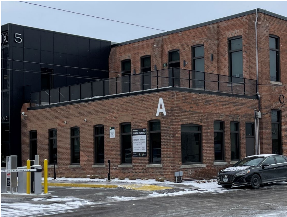
Figure 22. View of the north and west elevations of the one-storey north wing of the Office and Aqua Ammonia Building, featuring segmental arched window and door openings with brick voussoirs (Heritage Planning, 2025).
