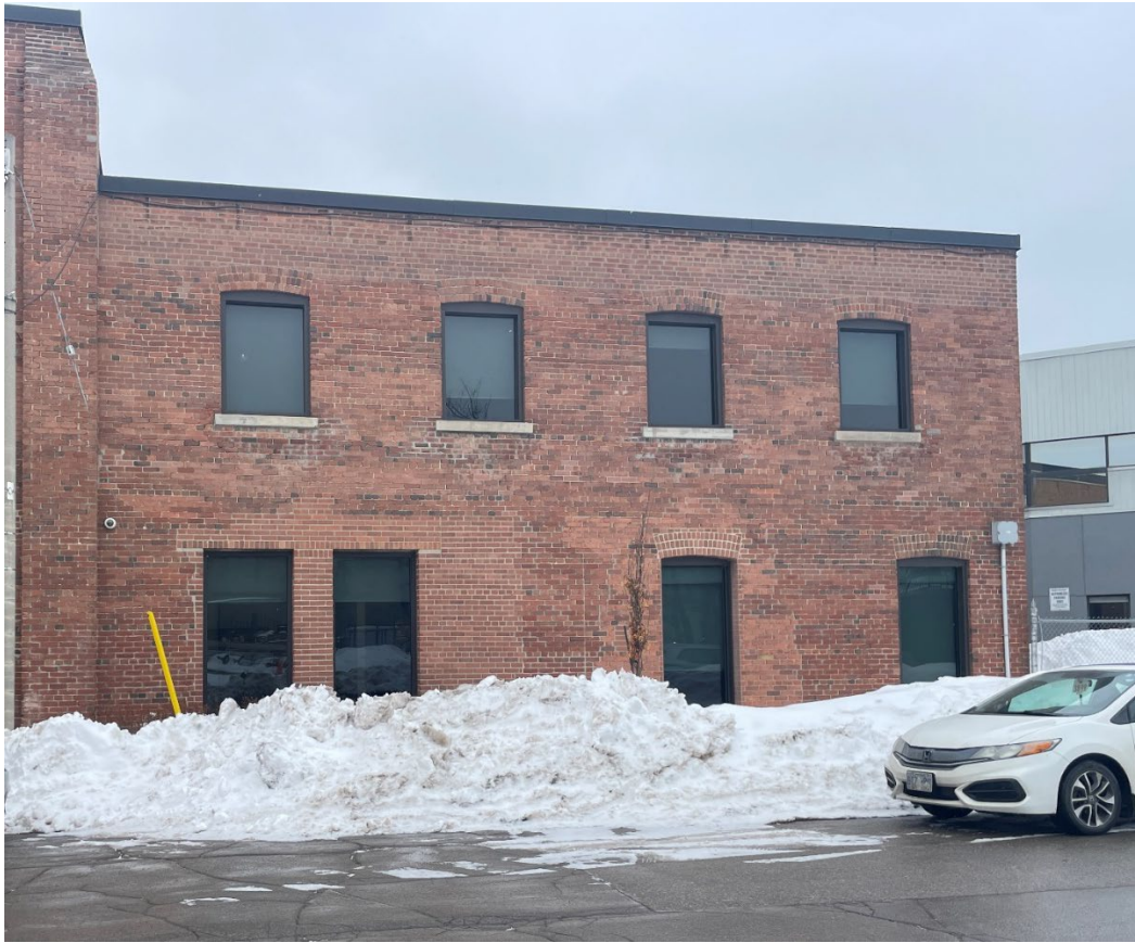
Figure 20. View of the west elevation of the south wing which features four asymmetrical placed window openings at the first storey with the northerly two featuring flat headed openings while the southerly two feature segmental arch openings with brick voussoirs (Heritage Planning, 2026).
