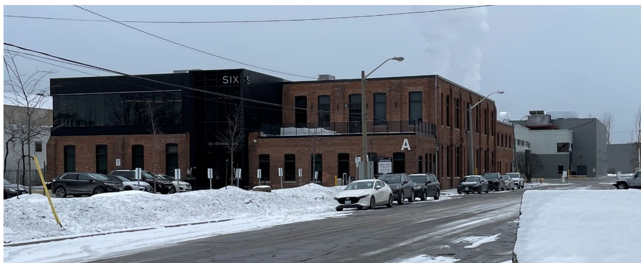
Figure 3. The main (north and west) elevations of 65 Heward Avenue (Heritage Planning, 2026).
