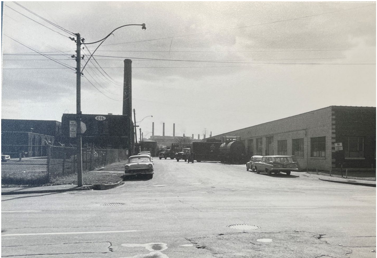
Figure 13. 1961 archival image looking south from Eastern Avenue towards Heward Avenue, showing the "CIL", Canadian Industries Limited, logo on the north elevation of 65 Heward Avenue (CTA).
