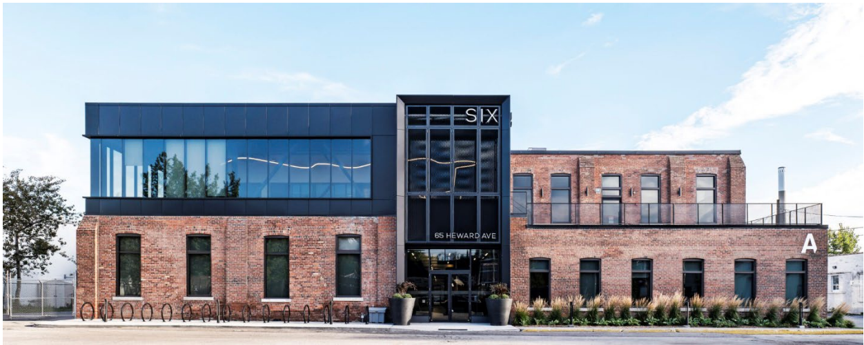
Figure 16. Image showing the extension completed by Cumulus Architects (Cumulus Architects).
