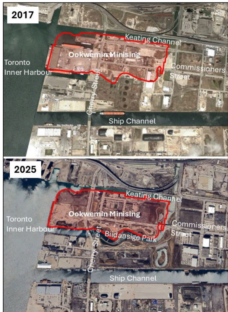
Figure 1. Ookwemin Minising was created between 2017 and 2024 as part of the Port Lands Flood Protection Project
